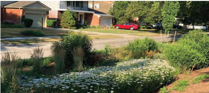
**Bioswales** are linear, planted channels that run along roads, parking lots, and/or sidewalks and provide a natural conveyance channel for stormwater runoff. Because they are planted (rather than concrete or pipe), they allow for natural infiltration of the stormwater which slows the velocity and improves the quality of the water that ultimately enters gray infrastructure systems.
