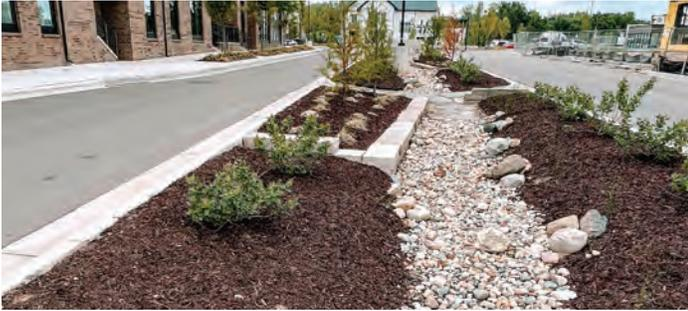
**Rain gardens** are shallow spaces below the existing grade that are lined with rock or other permeable substrate and planted with water tolerant plants. They collect precipitation or runoff from impervious surfaces and provide slower infiltration and filtration of the water to the ground below. Rain gardens can be connected to storm/sewer systems but are usually designed to hold and infiltrate stormwater within a few days.
