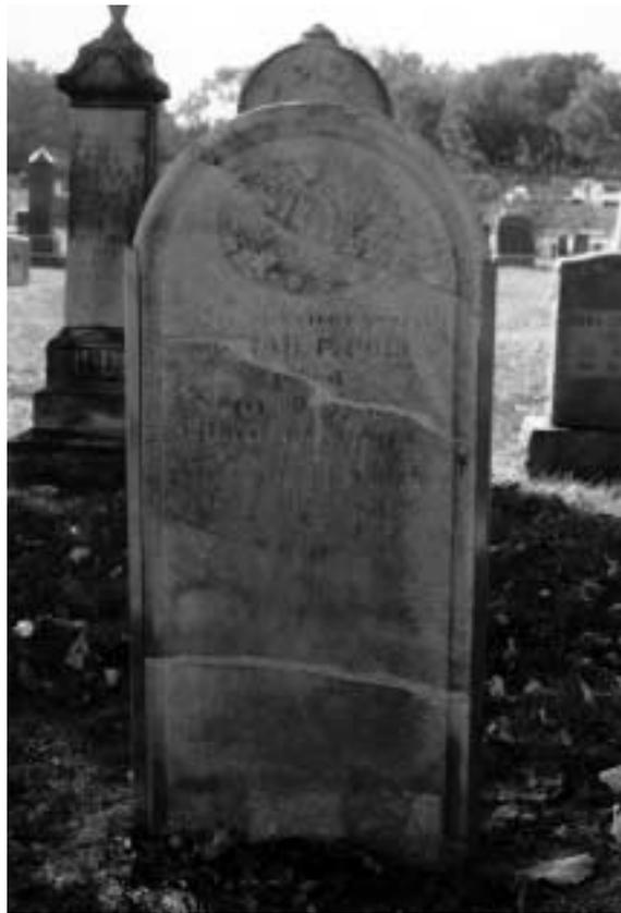
Professional conservators have in unique situations, girdled a marker with stainless steel channel. Here the repair is not easily seen and has not compromised the stone.
