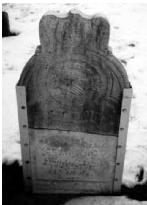
Drilling through a marker to affix braces is never an acceptable alternative.
