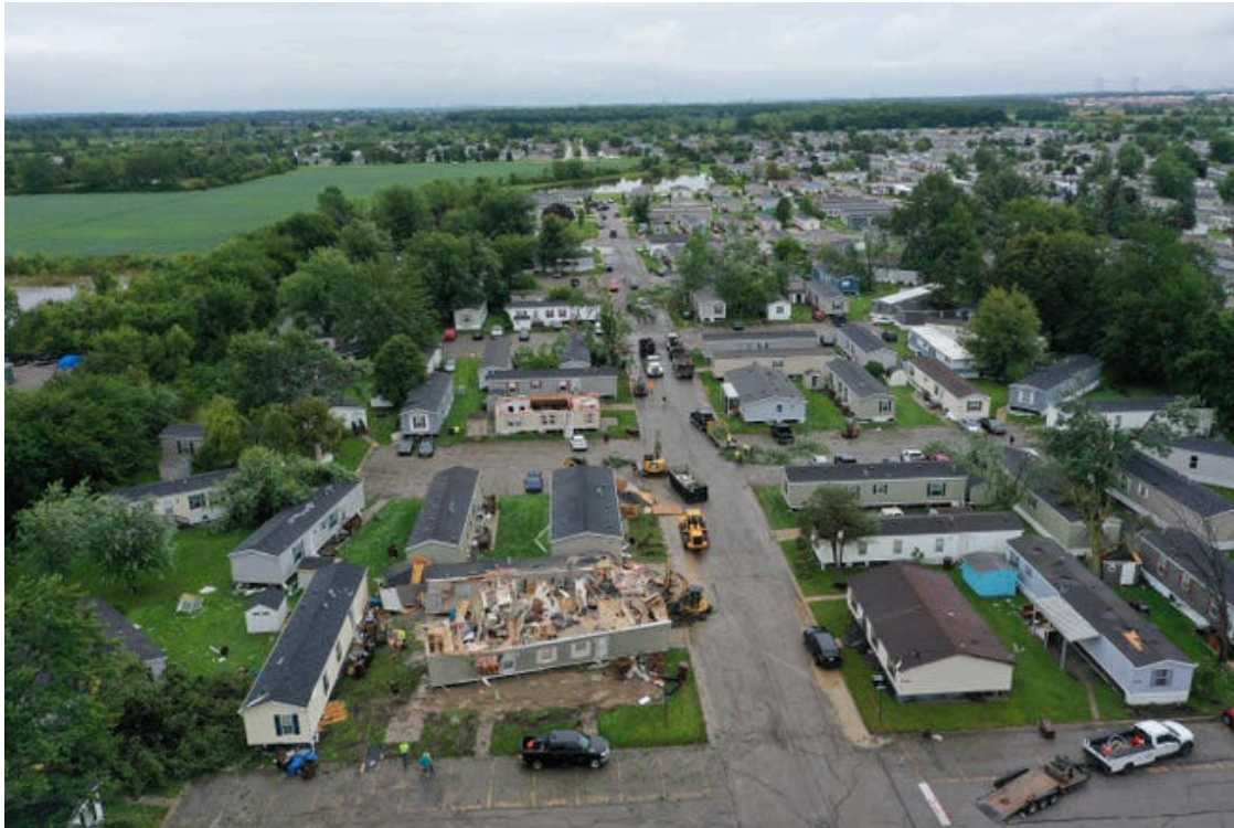
Figure 3: Mobile Home Park Tornado Damage
