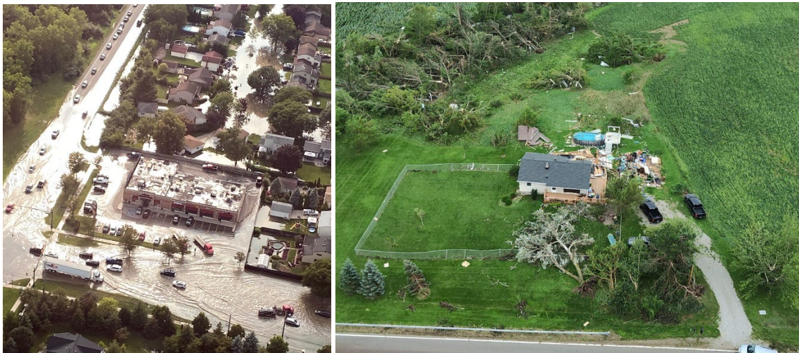
Figure 2: Flood and Tornado Damage
