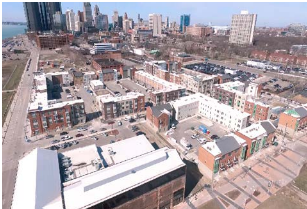
Orleans Landing Redevelopment – City of Detroit
