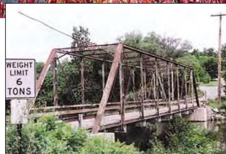
By late 1999, due to the structural deterioration of the bridge and concern for public safety, a reduced limit of 6 tons was imposed on the bridge. The Washtenaw County Road Commission began looking for funding to replace the bridge in early 2000. Concerned about preserving the historic bridge while retaining its rural character, and realizing that something needed to be done soon, local citizens formed the Citizens for Foster Road Bridge Conservancy (CFBC).
