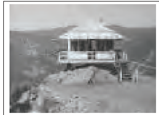
Figure 5: Jones Point Fire Lookout Tower, Groveland Ranger District, Stanislaus National Forest, CA, about 1954. From website: fs.usda.gov/wps/portal/fsinternet .
