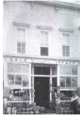
Figure 6: Growing American demand for retail goods gave birth to the commercial storefront, a new architectural form. The narrow buildings with their large front windows and central doors provided
