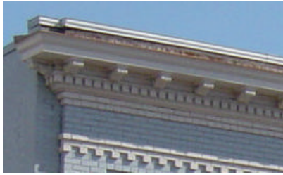
Figure 37: Cornice: The exterior trim of a structure at the meeting of the roof and wall.
