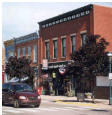
Figures 15 & 16: Improvements in the manufacture of structural steel members allowed wider openings between walls.
