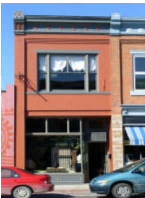
Figures 15 & 16: Improvements in the manufacture of structural steel members allowed wider openings between walls.
