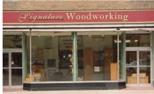
Figures 11 & 12: As American manufacturers learned to make larger sheets of glass, or plate glass, display windows grew larger, occupied more of the storefront, and offered unobstructed views of merchandise.
