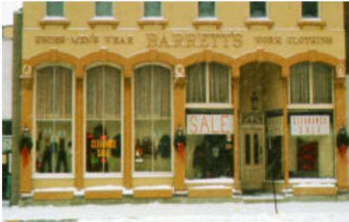
Figures 11 & 12: As American manufacturers learned to make larger sheets of glass, or plate glass, display windows grew larger, occupied more of the storefront, and offered unobstructed views of merchandise.
