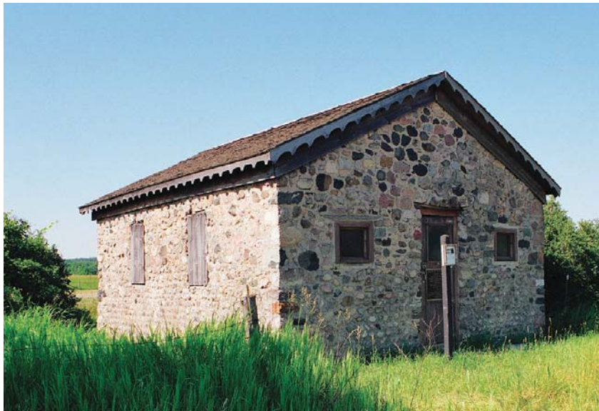
The 1847 Sessions School in Ionia County is one of the earliest remaining primary district school buildings in the state and displays unusual cobblestone construction. It was used for 50 years as a school; many primary district school buildings served for even longer periods of time.
