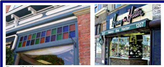
Figures 17 & 18: Structural pigmented glass, aluminum, and neon lighting made new details possible.
