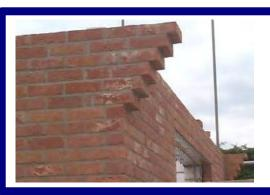
Figure 44: Rooflines are often embellished with cornices or other decorative details including arched or **stepped sections**.
