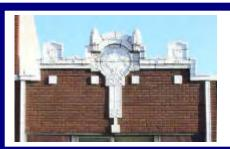
Figure 40: Cornices can also be constructed of other materials. The example here is terra cotta.
