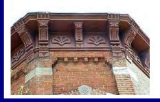
Figure 39: A pressed metal cornice conceals the roofline of this building.
