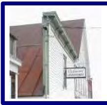
Figure 43: If the vertical extension is great, perhaps doubling the height of the building, it is known as a **false front**.
