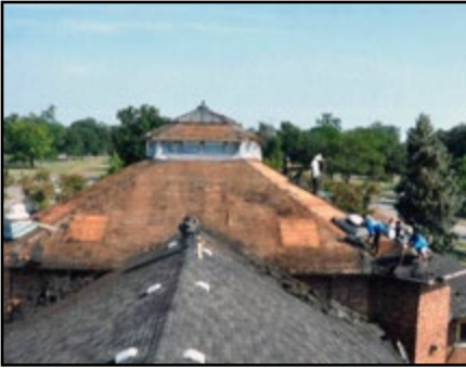
Belle Isle Aquarium roof rehabilitation, Detroit. State Historic Preservation Office.
