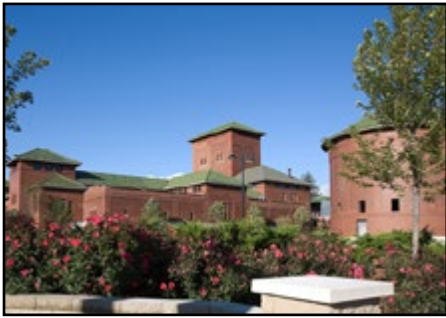
Water Filtration Plant, Grand Rapids. Photo: DeVries Companies.
