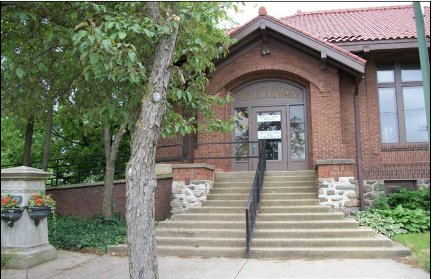
Allegan Library. State Historic Preservation Office
