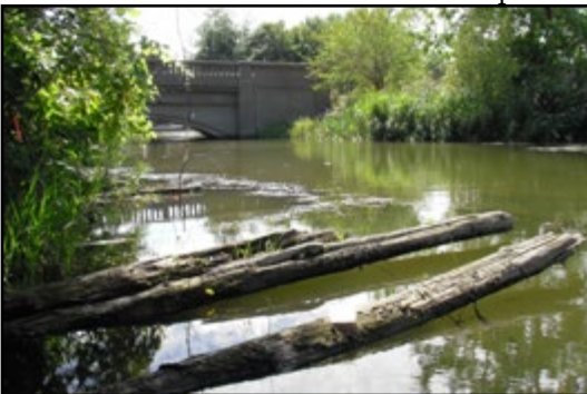
Hull's Trace North Huron River Corduroy Road Segment, Brownstown Township, Wayne County. Daniel Harrison, photographer.
