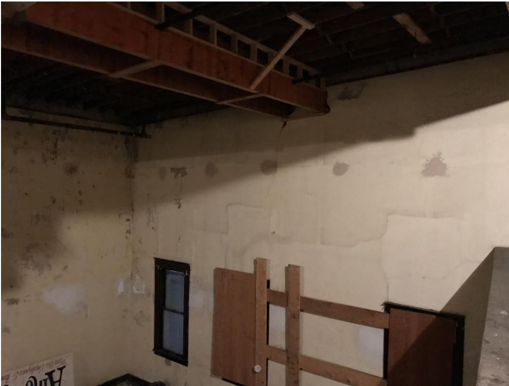
Photo 21: Gymnasium/Opera Hall Wall; Two sets of patches indicate anchorage locations
