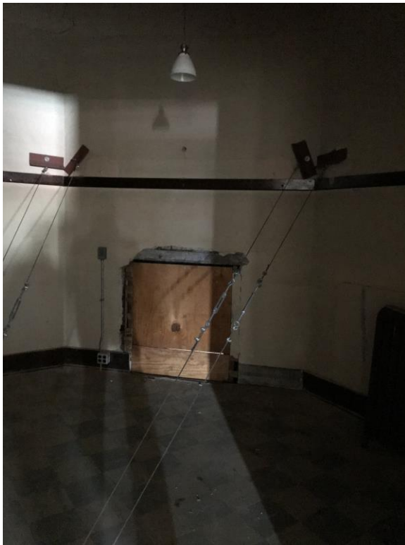
Photo 19: Cable restraints at Approximate Location of Façade Anchorage
