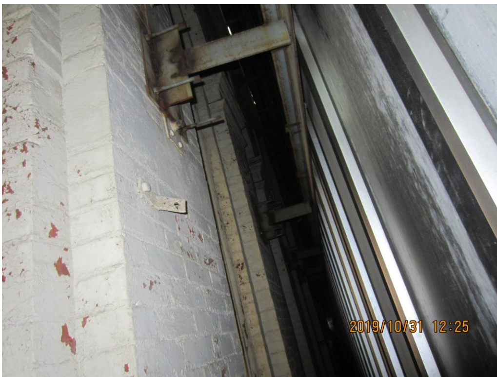
Photo 16: Façade Anchor at Mid-height of Third Floor
