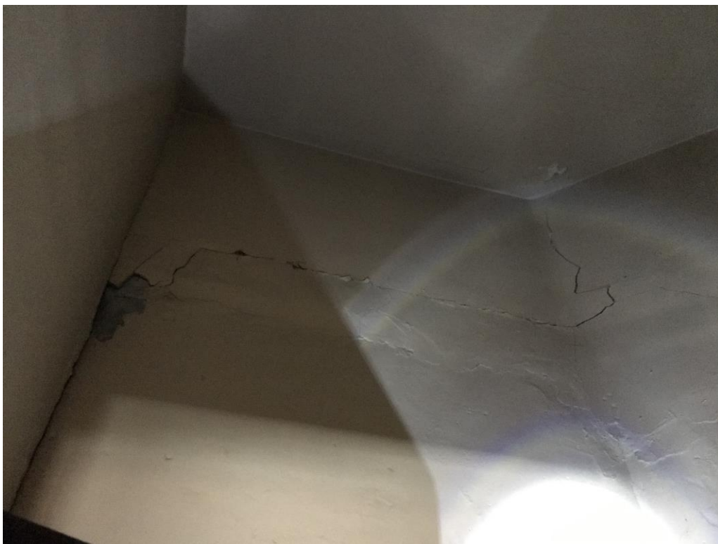
Photo 17: Damage to Existing Mass Masonry Exterior Bearing Wall
