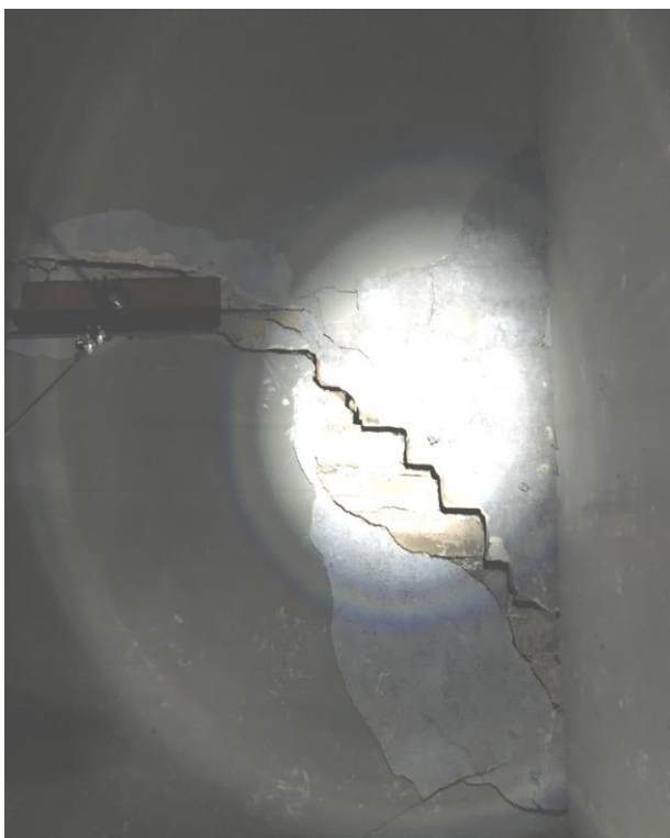
Photo 18: Damage to Existing Mass Masonry Exterior Bearing Wall
