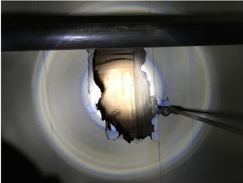
Photo 8: Wood Framing in Lot 5 Building Structure
