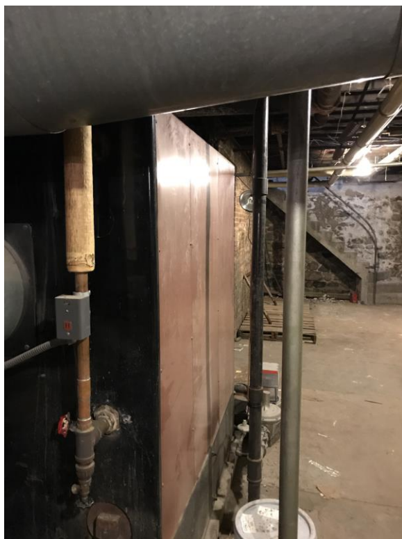
Photo 4: Shoring Posts in Basement
