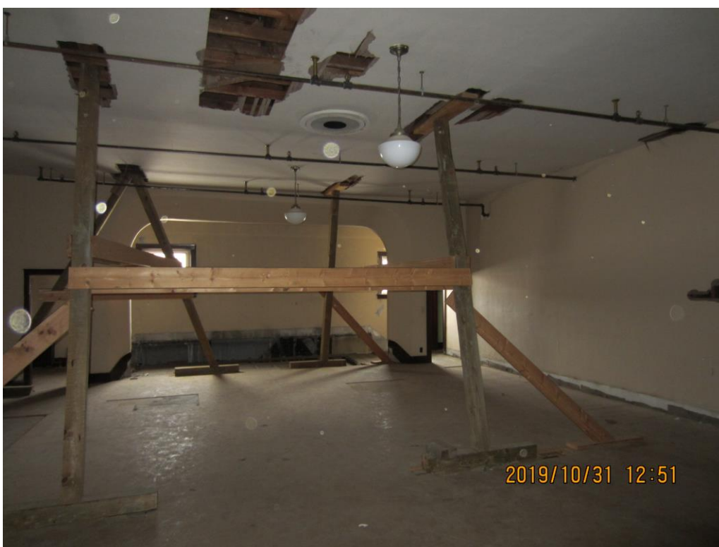
Photo 12: Supplemental Braces Supporting Roof Framing at Fraternal Hall
