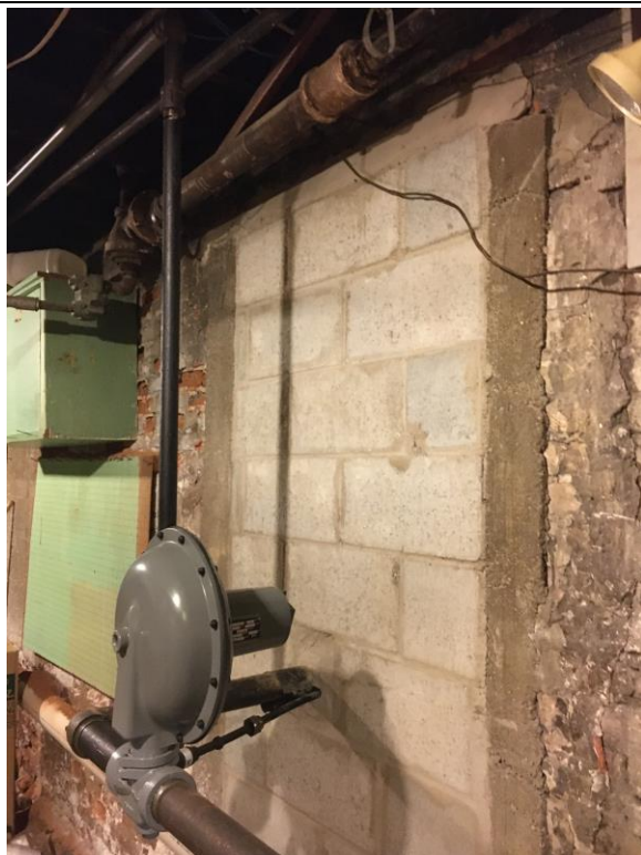
Photo 3: Concrete Masonry Wall Infill
