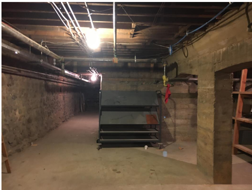
Photo 2: Stone Bearing Walls and Concrete Arched Wall
