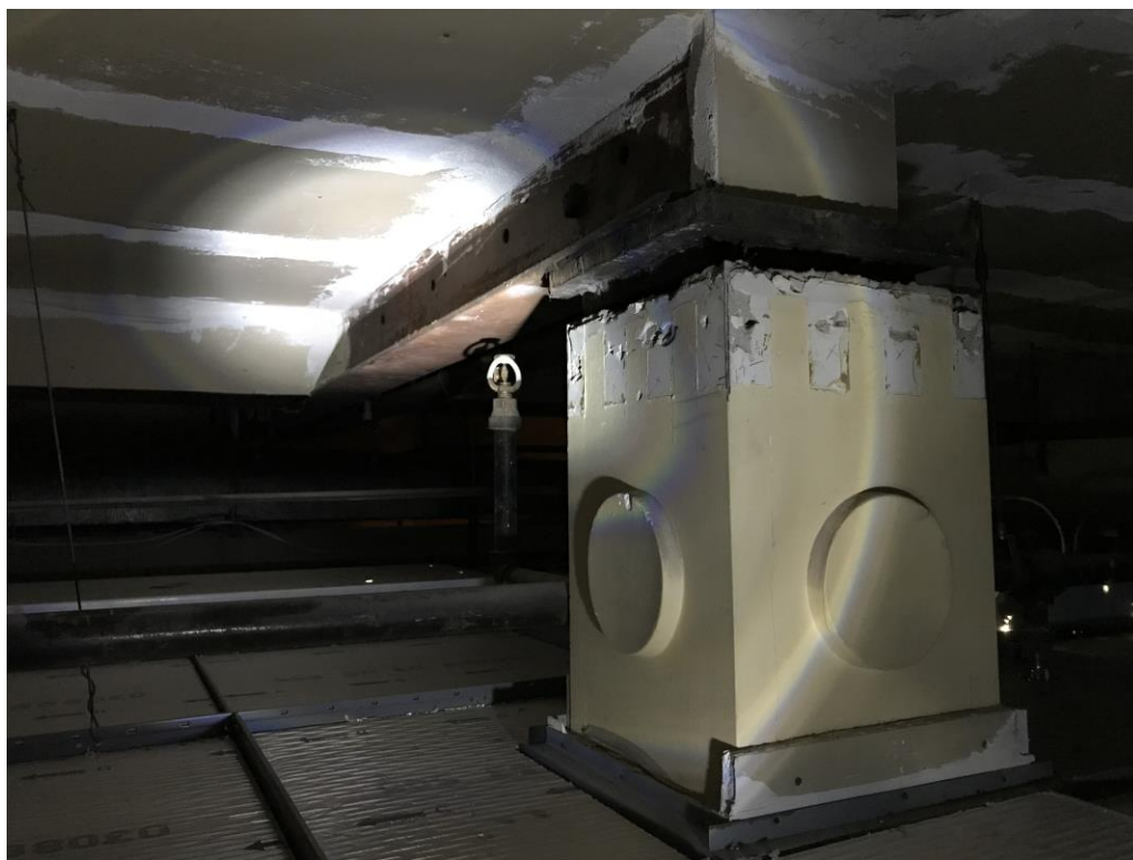
Photo 7: Higher Hard Ceiling, Steel Transfer Framing, and Column in Lot 6 Building Structure
