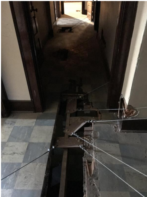
Photo 20: Cable restraints Anchored to Third Floor Framing
