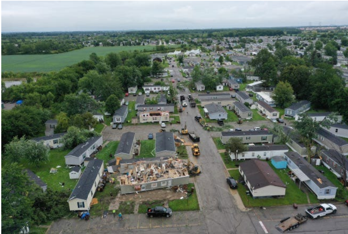
Figure 3: Mobile Home Park Tornado Damage
