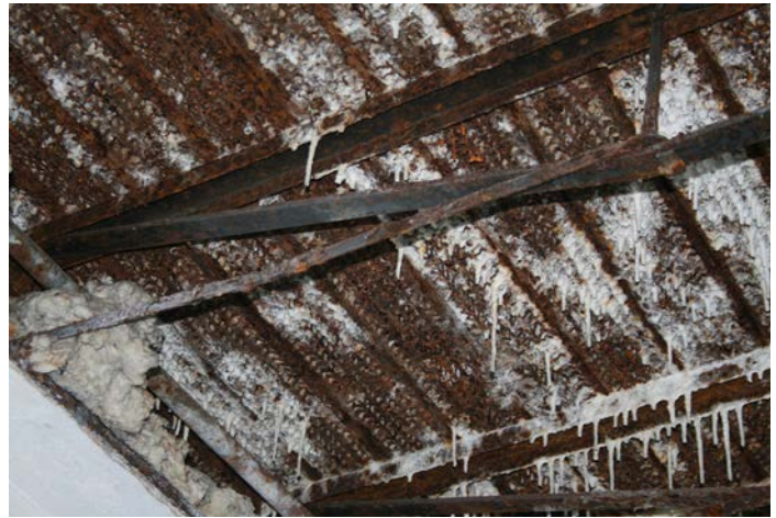
Figure 1D-50 Corroded and warped brace between top of interior wall and bar joist bottom chord.
