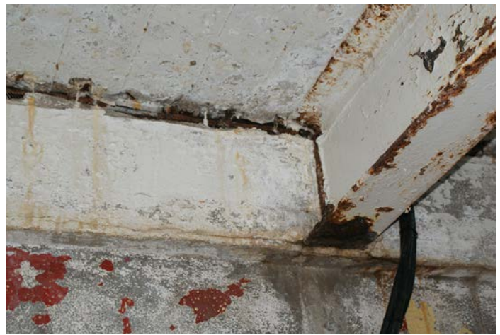
Figure 1D-224 Poor condition of exposed steel beams and concrete surfaces on Level 5.
