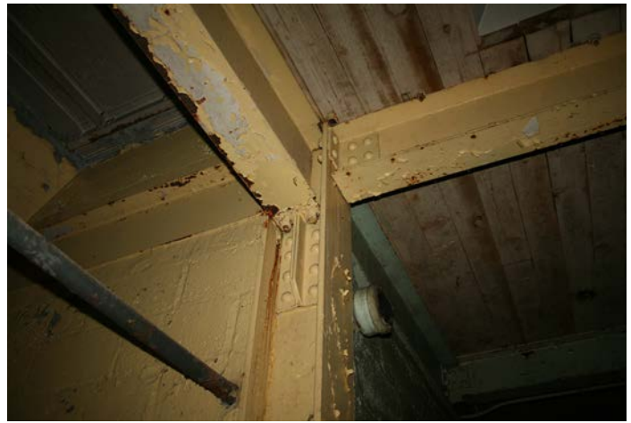
Figure 1D-36 Typical steel beam to column connections exposed in basement of pier deck, Level L-1 floor structure.
