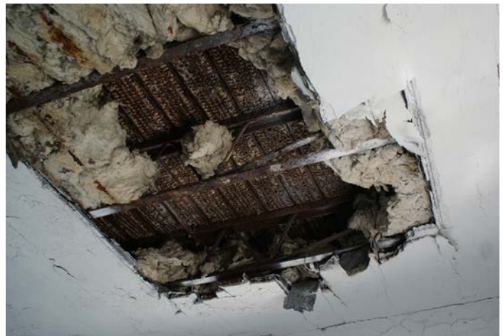
Figure 1D-190 Extreme damage of the plaster ceiling and metal lath in the Kitchen on Level 2.
