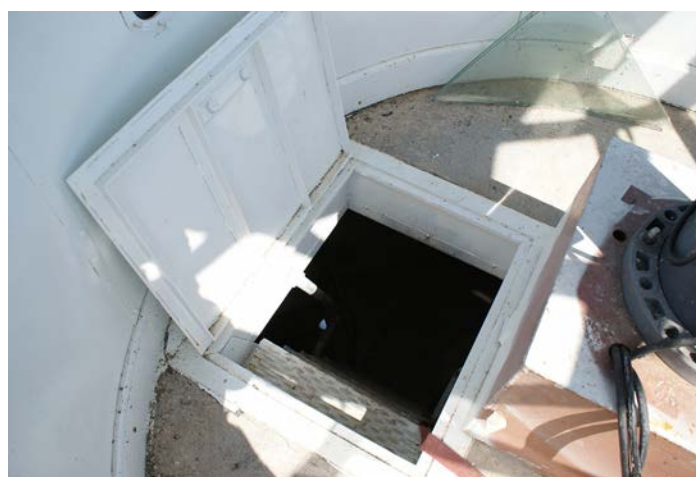
Figure 1D-123 Floor access hatch into the Lantern.
