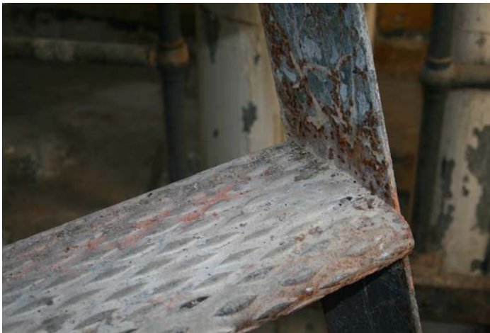
Figure 1D-60 Stair tread and plate stringer on ladder between Level L-5 and Level L-6.
