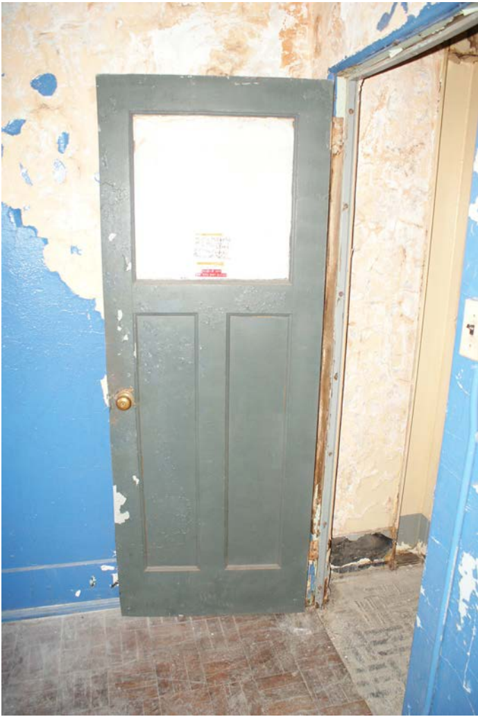
Figure 1D-196 Two-panel wood door with glass light at Office on Level 2.
