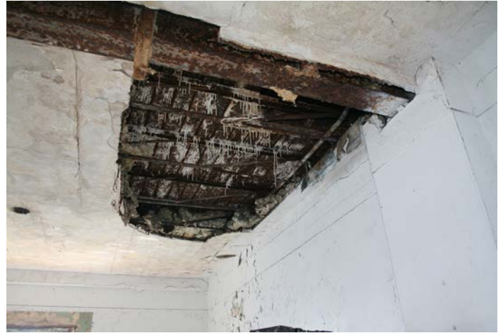
Figure 1D-46 Missing ceiling finish below watch deck, Level L-3, structure. Note stalactites forming on steel bar joist surfaces.
