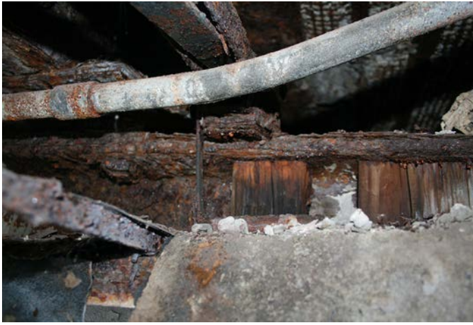
Figure 1D-51 Corroded joist bearing seat and flanges of steel support beam. Note water stained wood furring.
