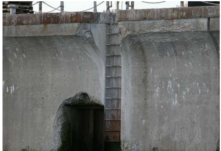
Figure 1D-06: Crazed cracking at the vertical and underside surfaces of the fluted edge of the concrete crib.
