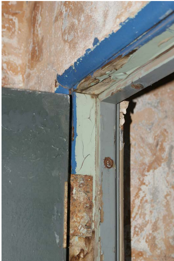
Figure 1D-202 Typical interior wood door frame on Level 2 with metal plaster stops.
