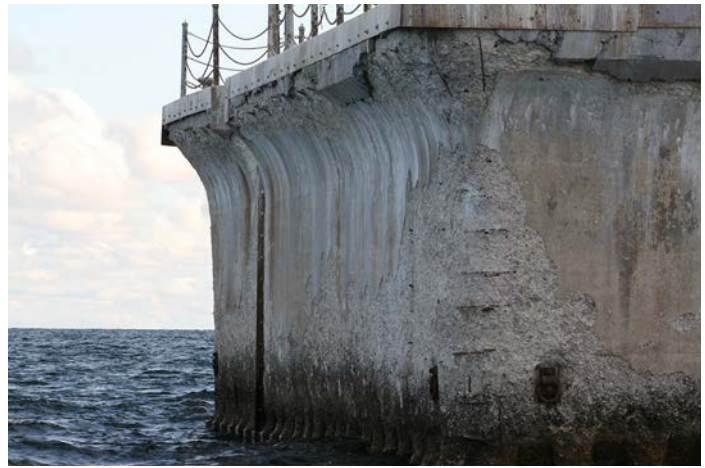
Figure 1D-05: Spalling over large areas of the concrete crib exposing reinforcing bars. Note the fluted top edge of the crib and the turned down steel plate bolted to the vertical edge of the flute. The steel sheet piling is visible at the water line.
