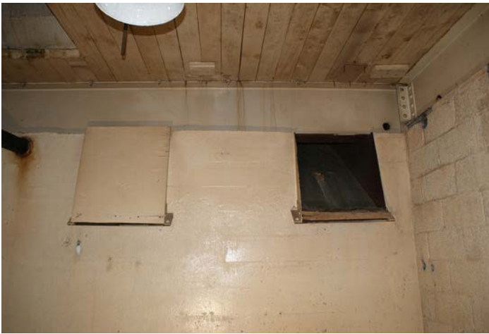
Figure 1D-159 View of the Coal Room and coal chutes.
