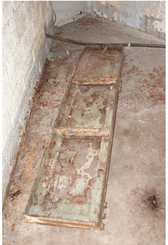
Figure 1D-109 Small door leaf of the sea door inside the basement.
