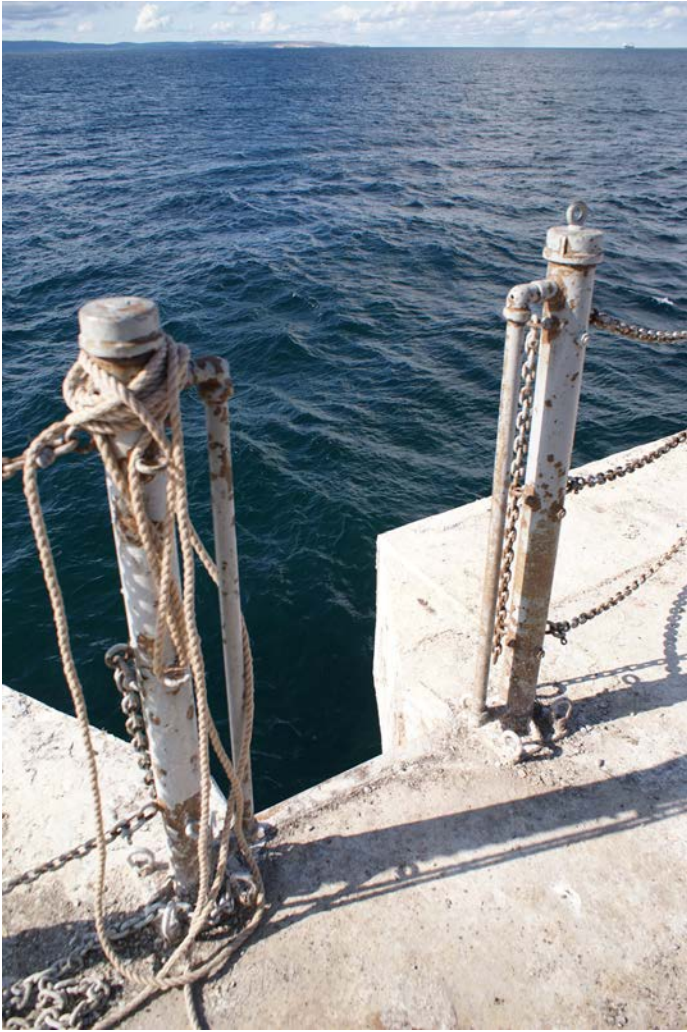
Figure 1D-84 Guardrail posts with hand-holds at one of the vertical ladders.
