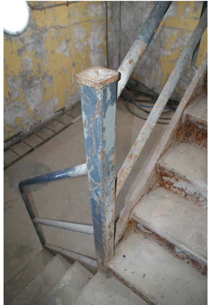
Figure 1D-217 Square steel newel post at Level 4.
