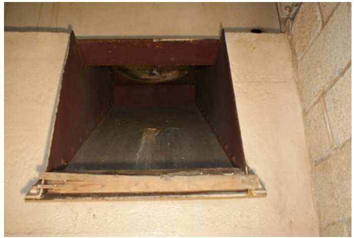
Figure 1D-160 View of a coal chute and partial view of the hatch cover at the Pier Deck.
