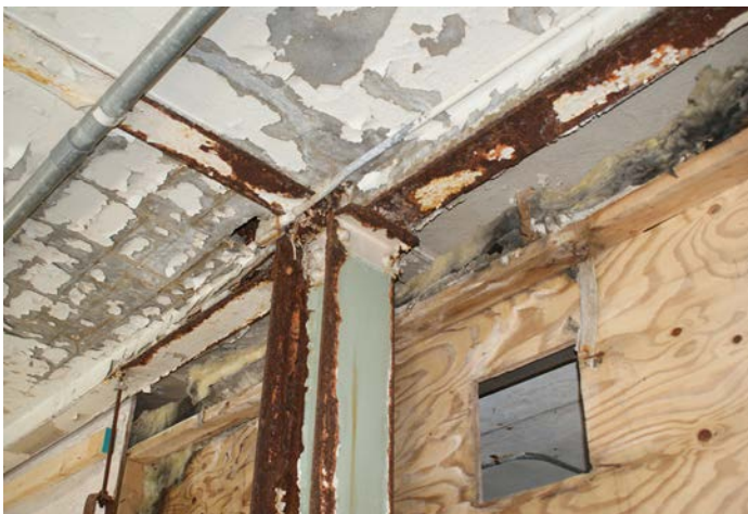
Figure 1D-183 Generally poor condition of interior paint and plaster finishes on Level 1.
