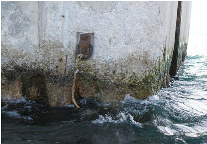
Figure 1D-73 Steel mooring anchors near the corner of the crib.
