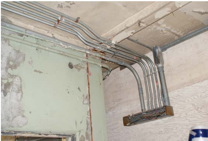
Figure 1D-231 Surface mounted electrical conduit on Level 1.
