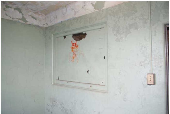
Figure 1D-199 Borrowed light in the Office wall.
