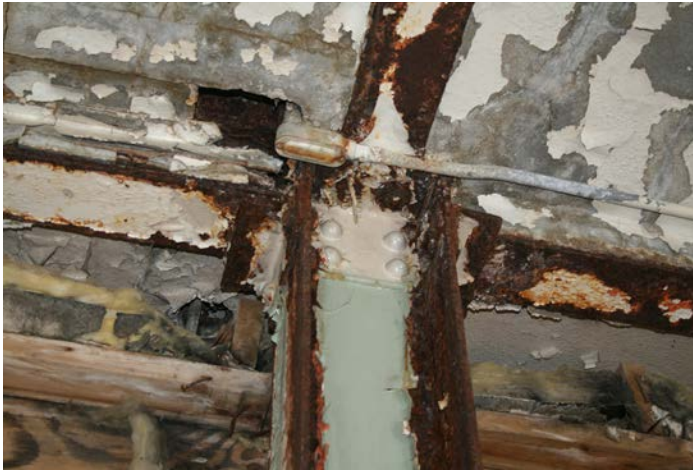
Figure 1D-39 Corrosion of steel framing members and connection at underside of second floor structure, Level L-2, at southernmost interior column.
