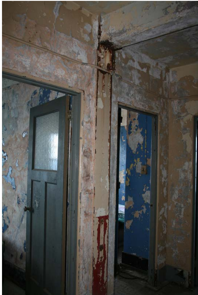
Figure 1D-27: Typical plaster finishes on interior, note painted steel column between doors.
