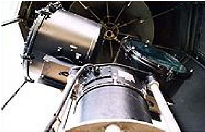
Figure 1A-09: Photo of the twin DCB-224 aero beacons with automatic bulb changers installed in the Pointe Aux Barques Lighthouse in the 1950s.
