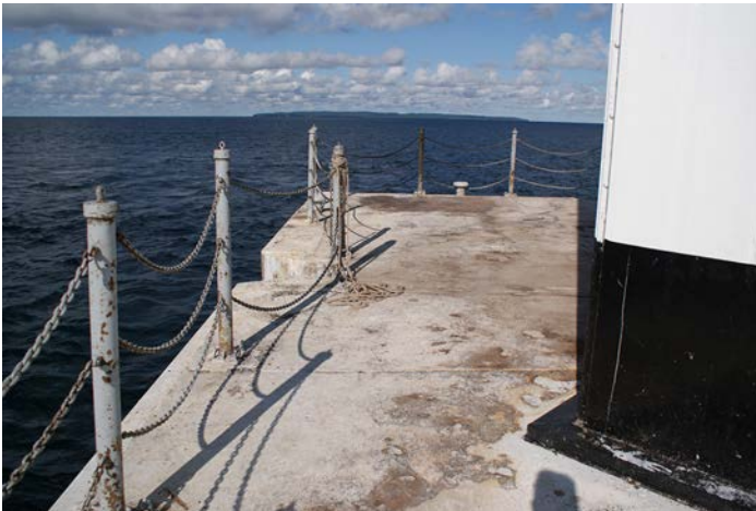
Figure 1D-81 Steel pipe posts and chain link guardrail at the perimeter of the Pier Deck.
