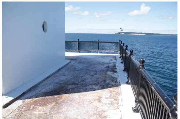
Figure 1D-89 View of the steel plate deck surface at the Watch Deck, Level 3.
