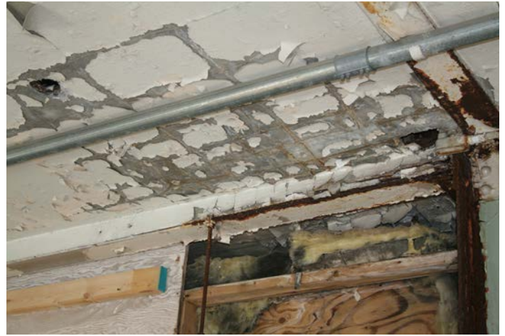
Figure 1D-30 Ghosting of metal lath through plaster ceiling. Note dark fiberglass insulation indicating potential water infiltration by boarded-up window.
