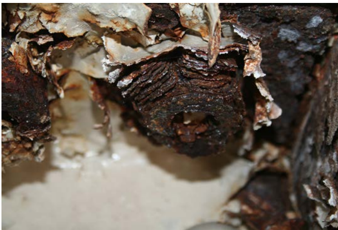
Figure 1D-41 Nearly full section loss of nut at through-bolt connection.
