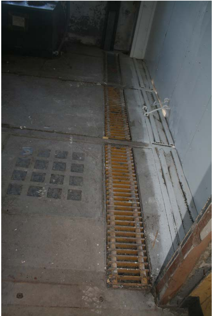
Figure 1D-26: Floor drains at boat room at pier deck, Level L-1.
