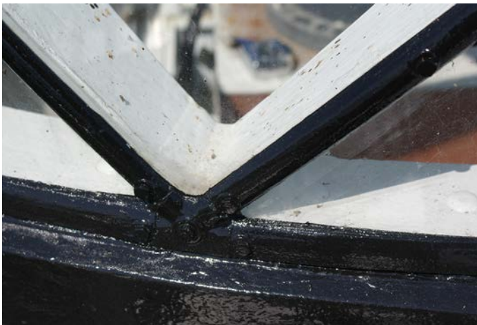
Figure 1D-130 Exterior view of glazing mullion covers.
