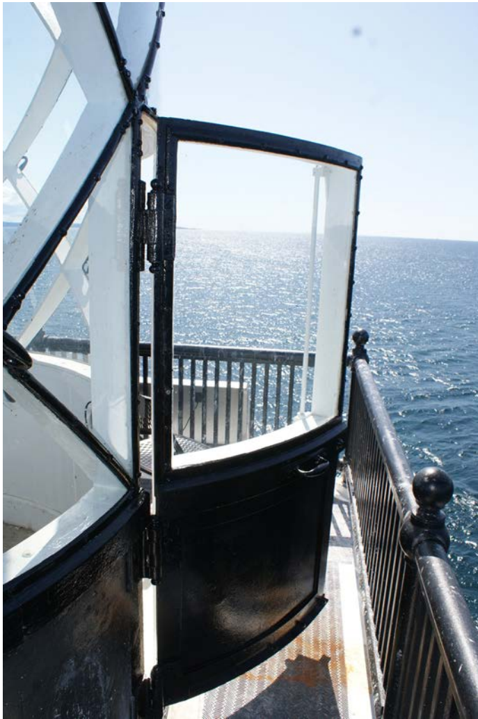
Figure 1D-137 Exterior view of metal door from Lantern to the Lantern Deck and metal guardrail.
