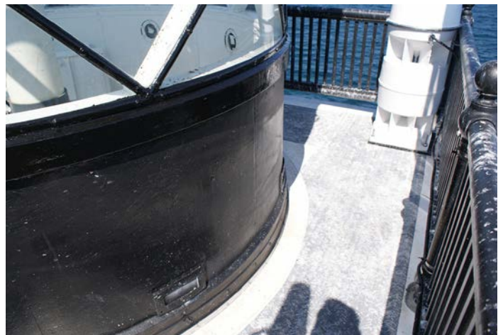
Figure 1D-139 EPDM membrane on the Lantern Deck surface.
