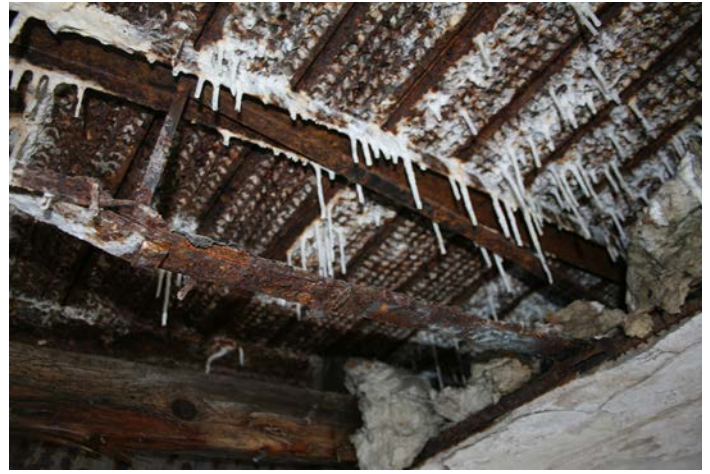
Figure 1D-52 Web member of steel bar joist is deformed, curved upward.
