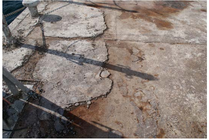
Figure 1D-78 View of the deteriorated surface of the steel plate on the Pier Deck.
