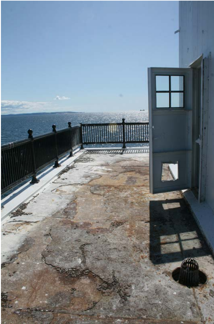
Figure 1D-15: Corroded steel plates on exterior surface of watch deck, Level L-3. Note roof drain at bottom right of photo.
