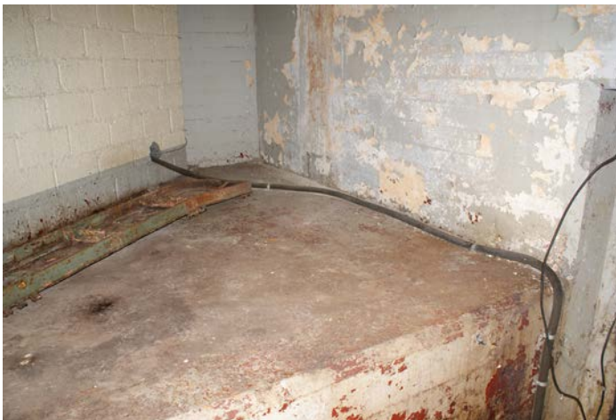
Figure 1D-226 Main electric cable secured to the Basement floor.
