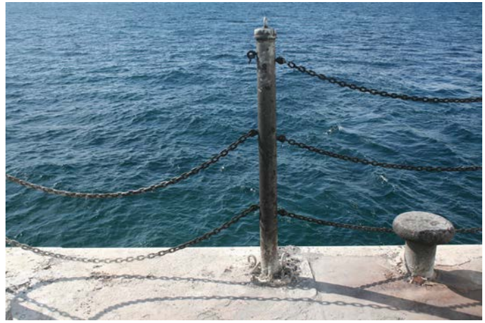
Figure 1D-09: Typical guard rail post. Note eye nuts for anchor bolts at base of column and base plate with vertical stiffeners. Note missing top chain on left side of post.
