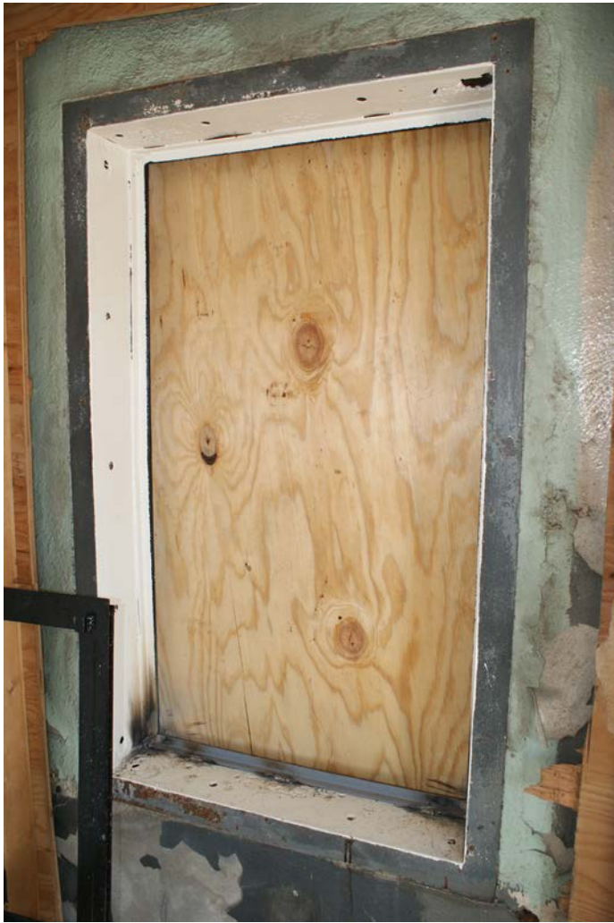
Figure 1D-101a Temporary plywood panel at a window opening.
