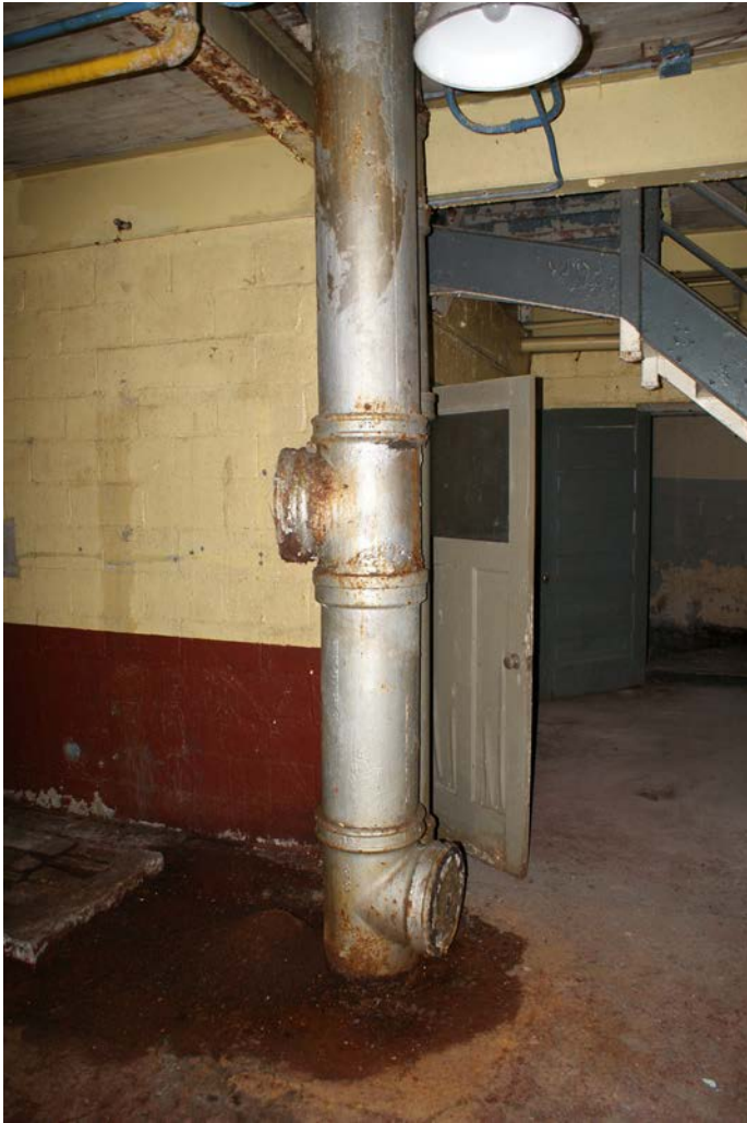
Figure 1D-241 Large chimney pipes located in the Basement.
