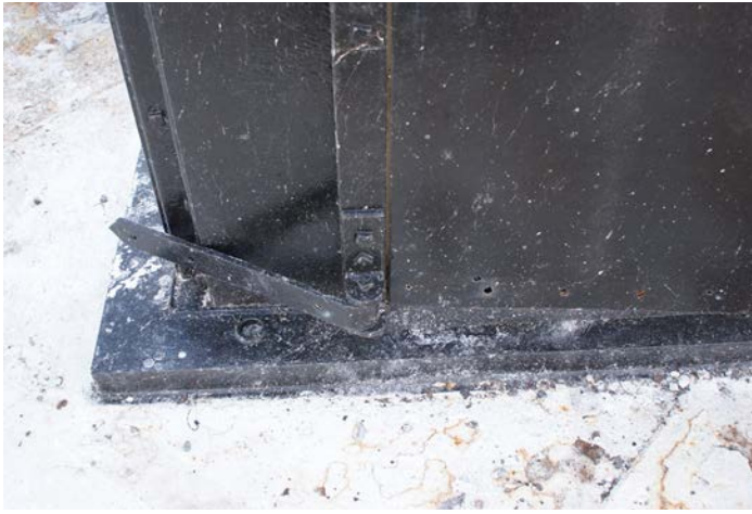
Figure 1D-116 Damaged strap hinge on the Boat Room doors, southwest wall.
