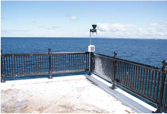
Figure 1D-90 Steel guardrail at the perimeter of the Watch Deck.
