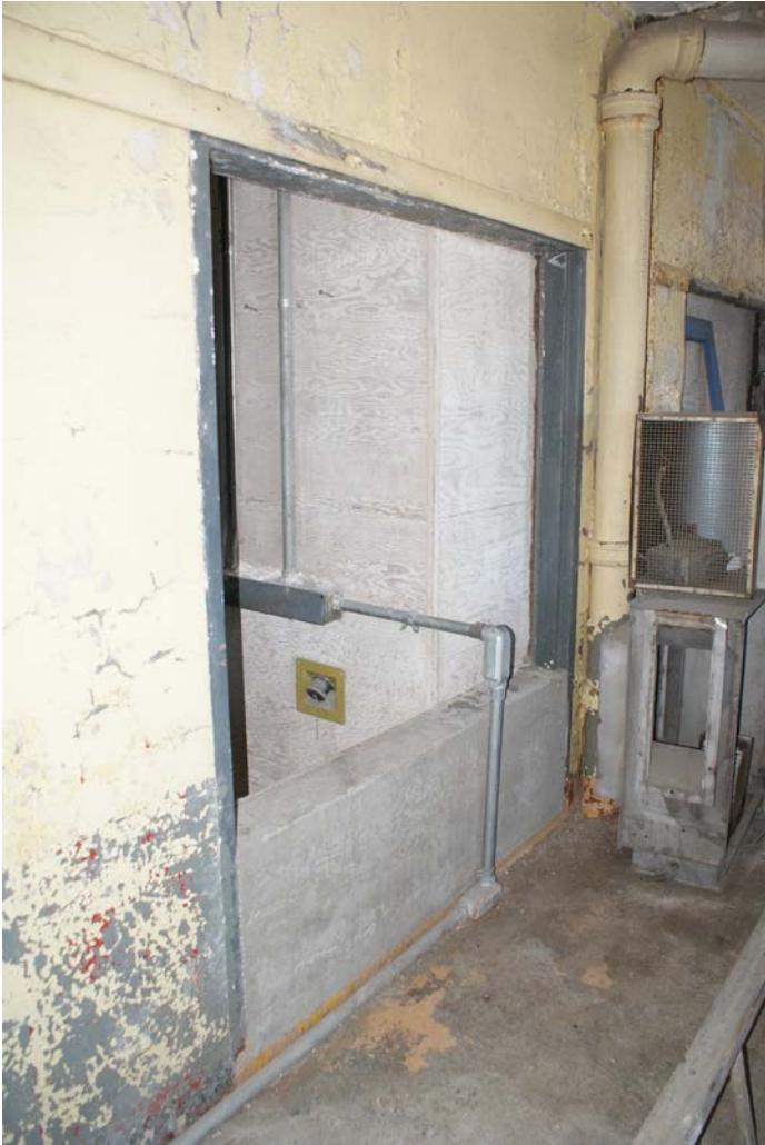
Figure 1D-169 Poured concrete containment wall across a door opening leading to the Boat Room.
