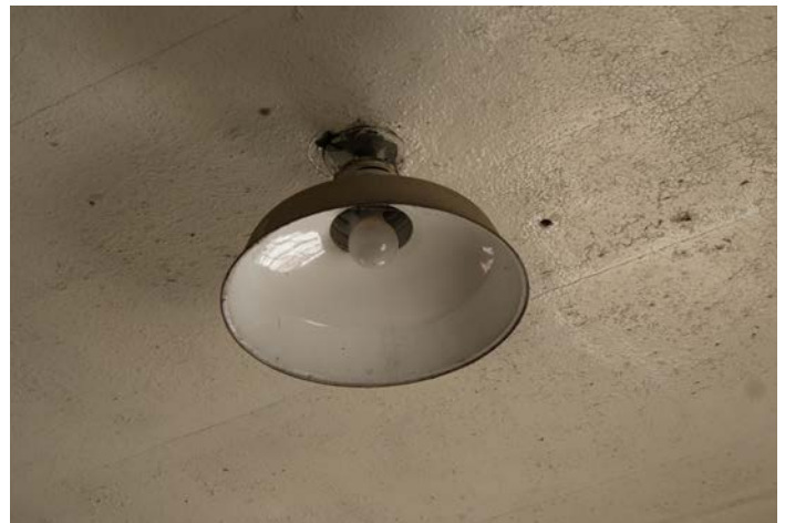
Figure 1D-235 Surface mounted incandescent light fixture.
