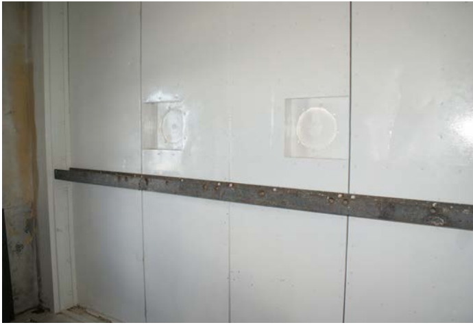
Figure 1D-113 Steel beam across the interior face of the Boat Room doors on the northeast wall.
