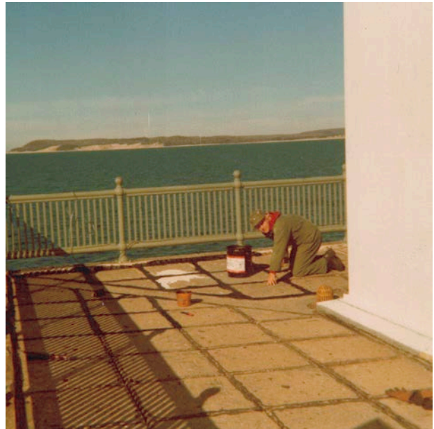
Figure 1B-66: Circa 1976-78 photo of a crewman sealing the joints in the concrete of the watch deck.
