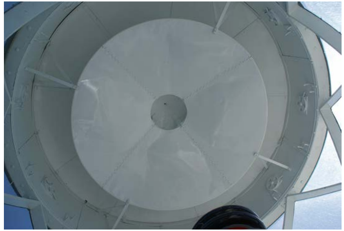
Figure 1D-125 View of the ceiling of the Lantern with the smoke shield intact.
