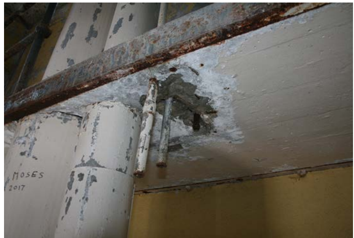
Figure 1D-56 Utility penetrations through concrete slab of floor structures of upper levels of tower.
