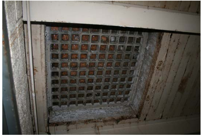
Figure 1D-34 Skylight in basement room ceiling in room for water level access door. Note cracking and deterioration of vertical edges of concrete at skylight opening.
