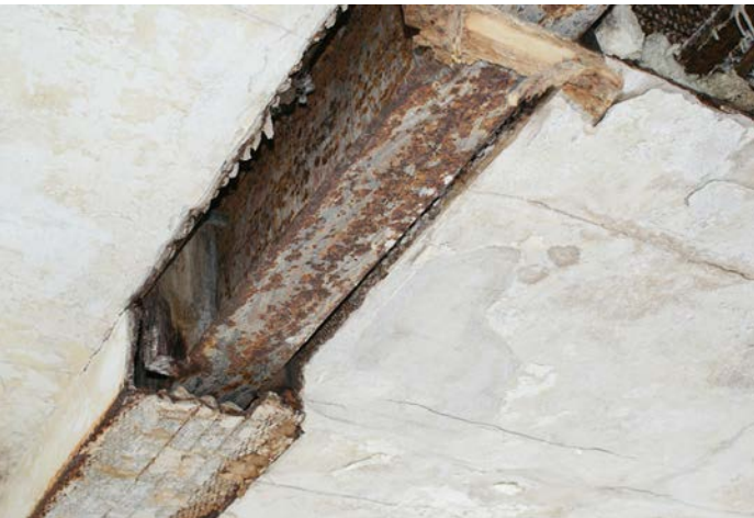
Figure 1D-207 Rusty steel beam and missing and damaged metal lath and plaster on Level 2.
