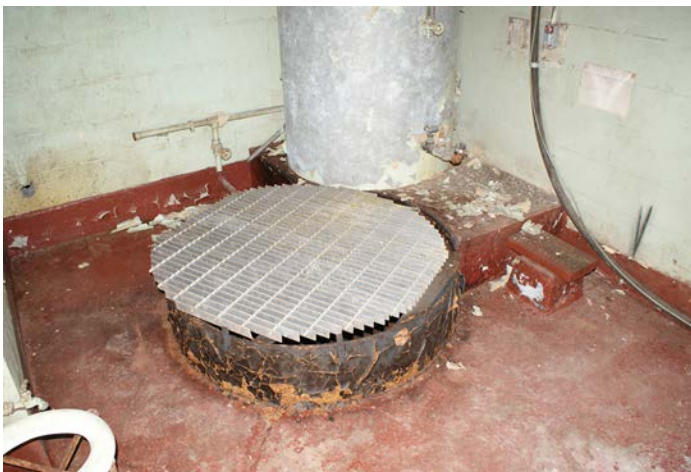
Figure 1D-153 Steel grate cover over the open water well in the Water Room.
