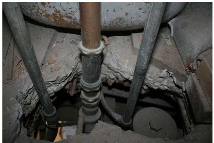
Figure 1D-42 Selective demolition of concrete slab at bathroom tub access. Embedded steel reinforcing bars are exposed at cut for utility penetration.
