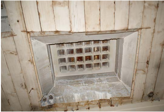
Figure 1D-163 Underside of a deck light as seen from the Basement.
