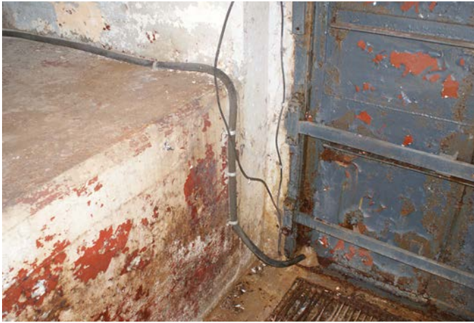
Figure 1D-225 Main electric cable entering the structure at the sea door in the Basement.
