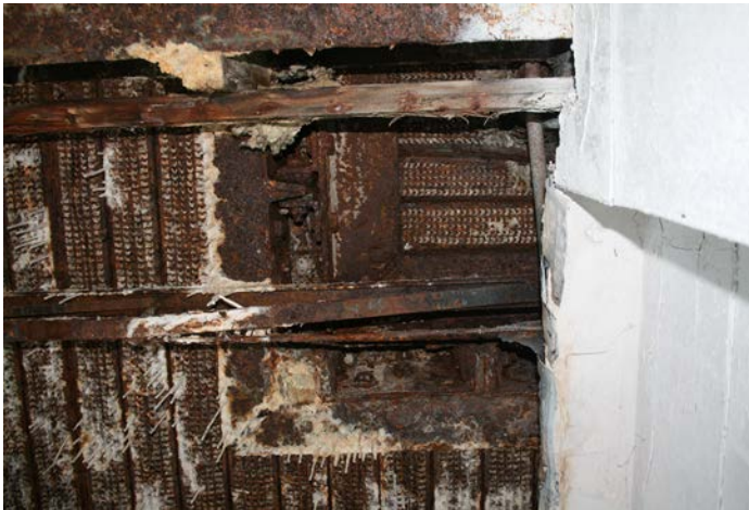
Figure 1D-53 Underside of upper tower wall framing bearing on watch deck, Level L-3, structure. Note water staining of wood furring, corrosion of steel, and stalactites.
