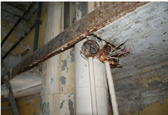
Figure 1D-219 Metal chimney pipes passing through Level 4.
