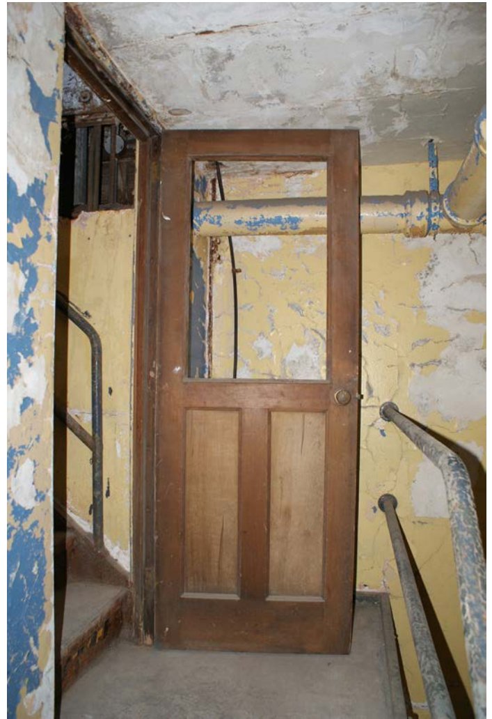
Figure 1D-210 Wood two-panel door with missing glass.
