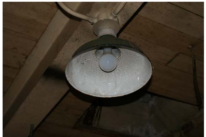
Figure 1D-236 Surface mounted incandescent light fixture.
