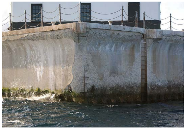
Figure 1D-69 Deteriorated concrete and exposed reinforcing bars on the northwest corner.
