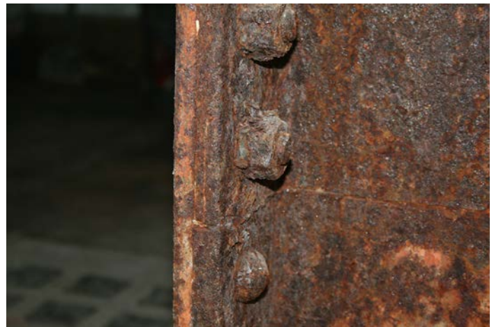
Figure 1D-38 Corrosion of nuts at through-bolt connection of column splice of southernmost interior column at pier deck, Level L-1.
