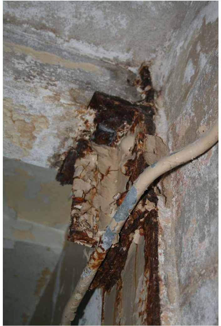
Figure 1D-44 Corroded steel connections of beam to column at watch deck, Level L-3, structure.
