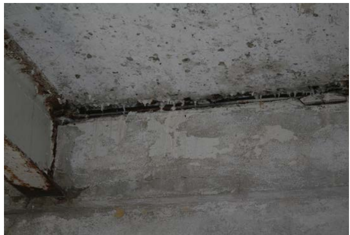
Figure 1D-57 Stalactites on underside of lantern deck concrete slab at perimeter of Level L-5.
