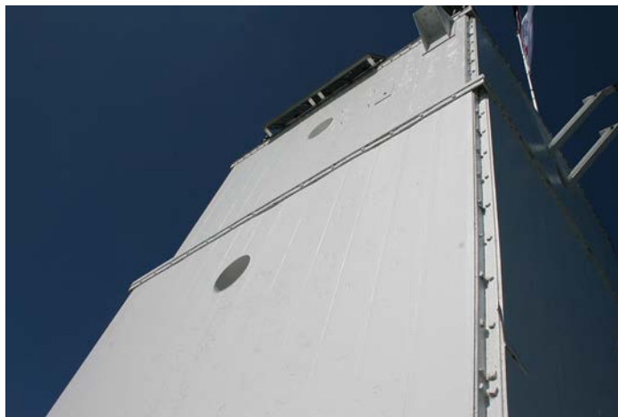
Figure 1D-12: Port style windows and corner angle connections of the upper portions of the tower wall assemblies.
