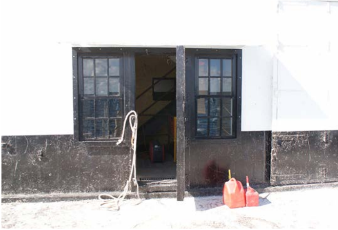
Figure 1D-102 Metal windows flanking the tower entry door at the Pier Deck.
