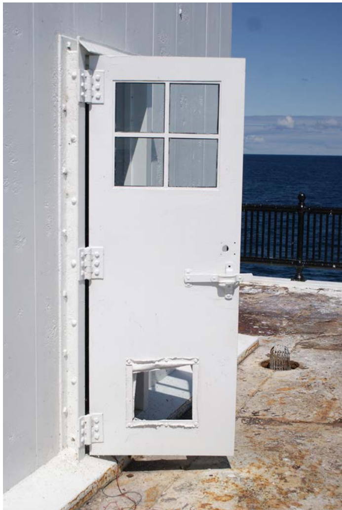
Figure 1D-118 Exterior metal door at the Watch Deck on Level 3.
