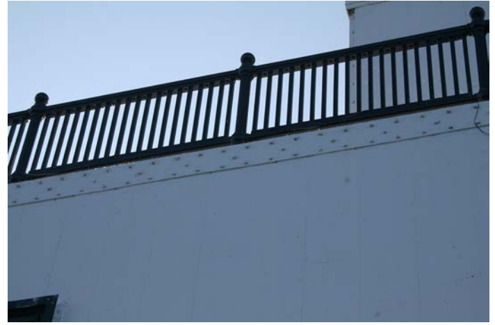
Figure 1D-16: Guard rail and bolted connection of turned down steel plate at edge of watch deck, Level L-3.
