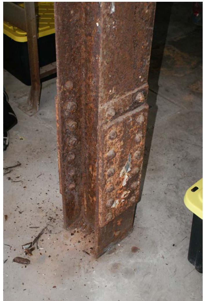
Figure 1D-182 Steel column on Level 1 with extreme rusted finish.
