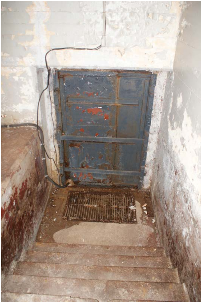
Figure 1D-106 View of landing and floor trench drain inside the sea door.
