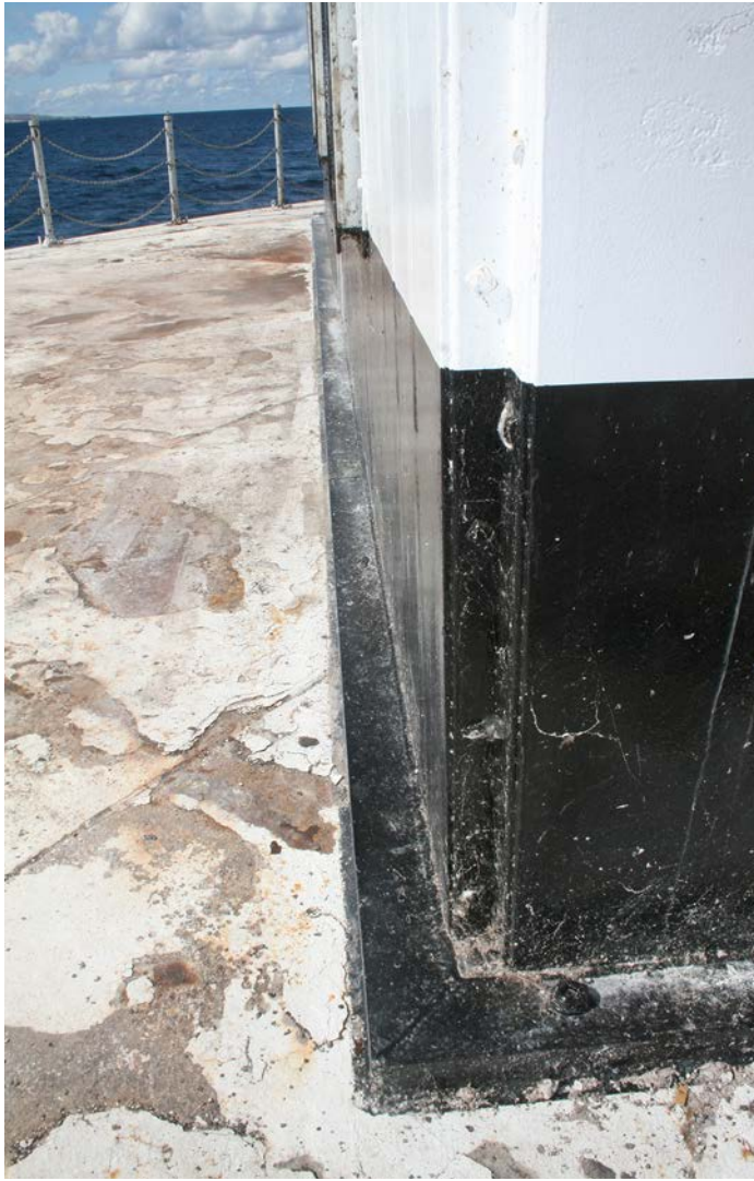
Figure 1D-10: Exterior curb between the pier deck, Level L-1, and the tower walls. Note single bolt of curb at the corner and the corner angle bolted to the end channels of each tower wall surface. The corroded steel plates on the deck surface are also visible.
