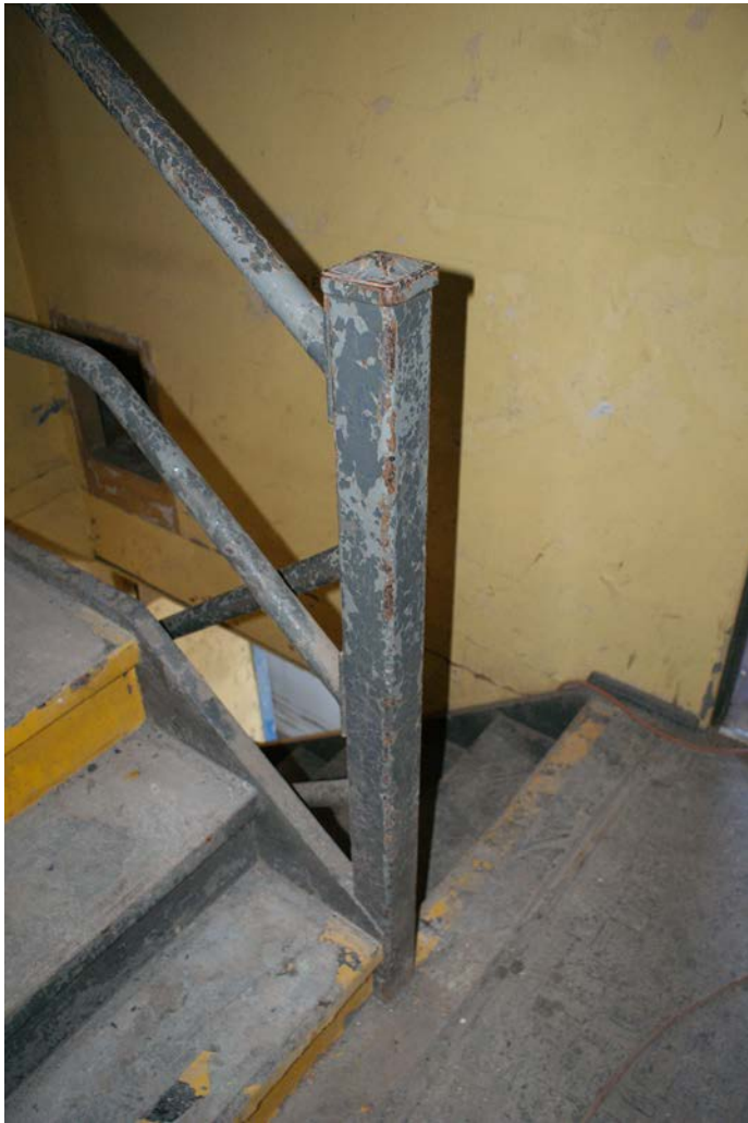
Figure 1D-186 Square steel newel post at Level 2.
