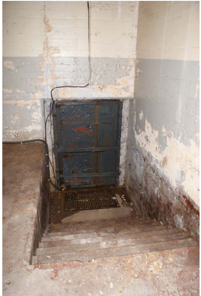
Figure 1D-105 Interior view of the metal sea door and interior concrete stair.
