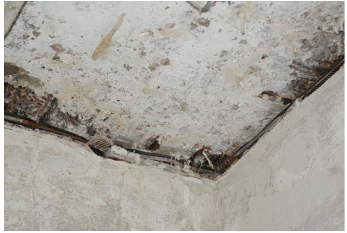
Figure 1D-223 Poor condition of exposed steel beams and concrete surfaces on Level 5.
