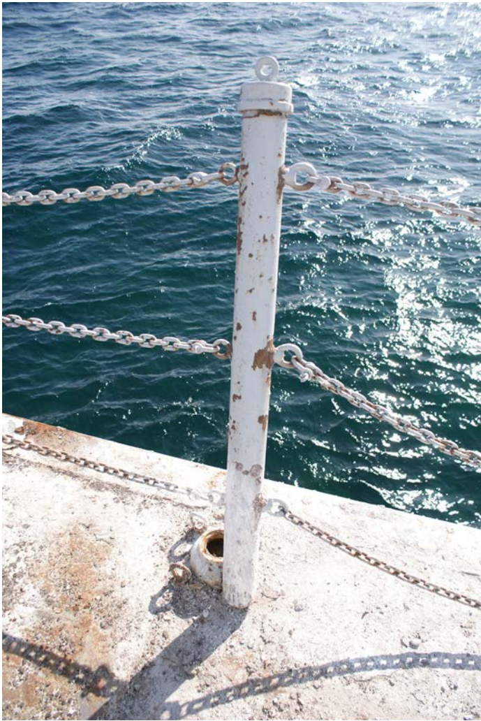
Figure 1D-82 View of damaged guardrail post broken from the base.
