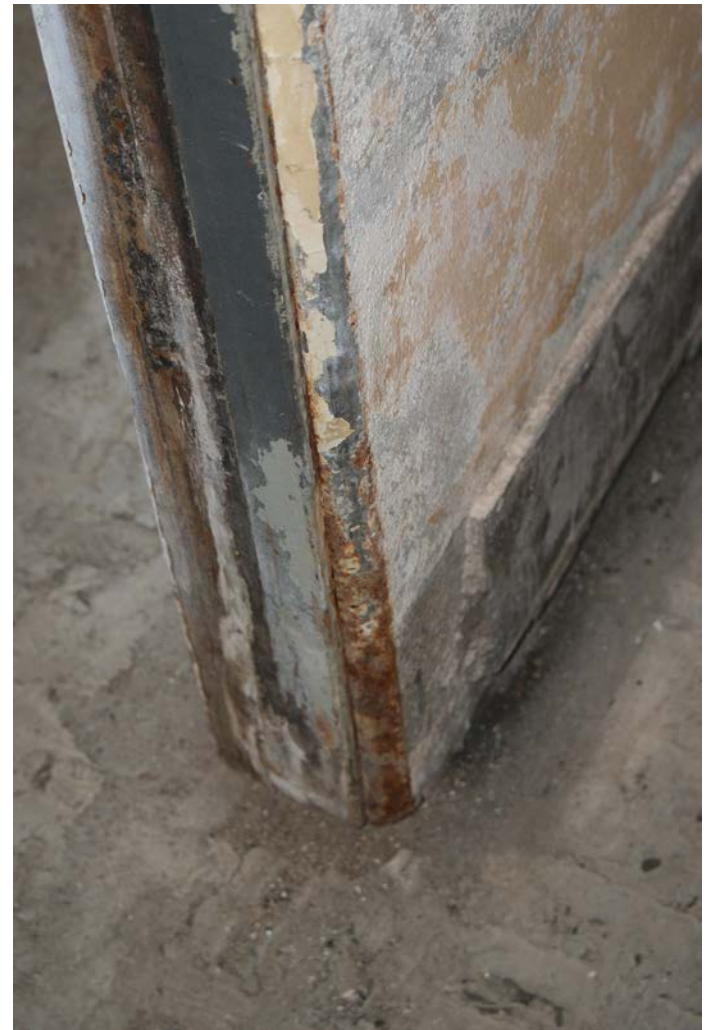
Figure 1D-203 Typical interior wood door frame on Level 2 with metal plaster stops.
