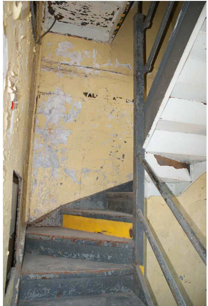
Figure 1D-185 Poor condition of interior finishes along with the winder style treads of the stair to Level 2.
