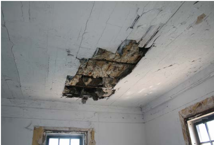
Figure 1D-45 Missing ceiling finish below watch deck, Level L-3, structure. Note insulation is tight to steel bar joists.
