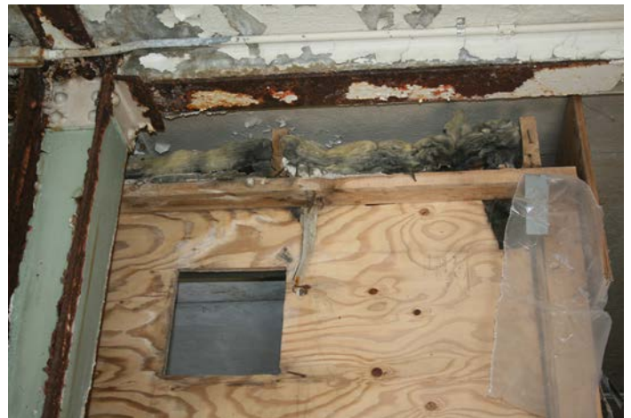
Figure 1D-32 Southern end of ceiling joists over equipment room that are supported on wood plate but wall studs are missing.
