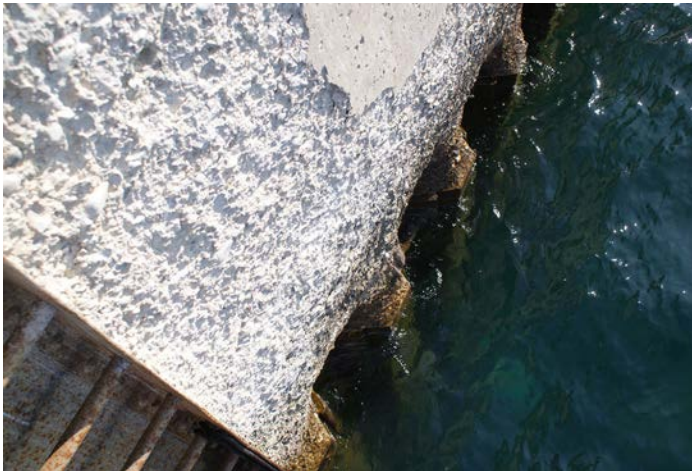
Figure 1D-65 Deteriorated concrete near the water surface above the steel sheet piling.
