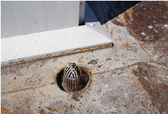
Figure 1D-94 One of two roof drains on the Watch Deck.
