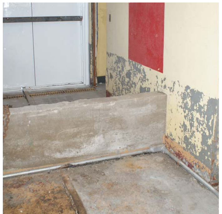
Figure 1D-168 Poured concrete containment wall in the Boat Room.
