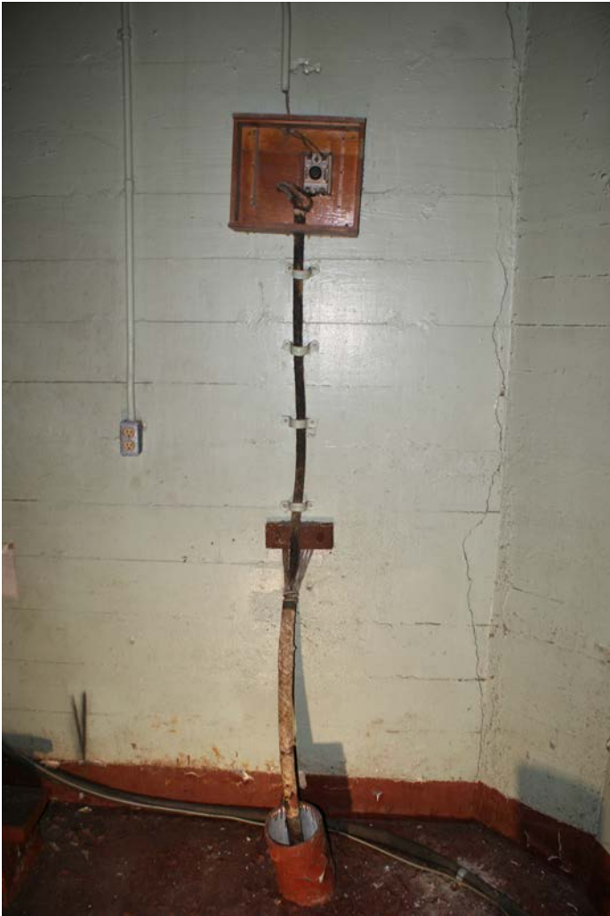
Figure 1D-237 Wiring in Basement Water Room from telegraph signaling system.
