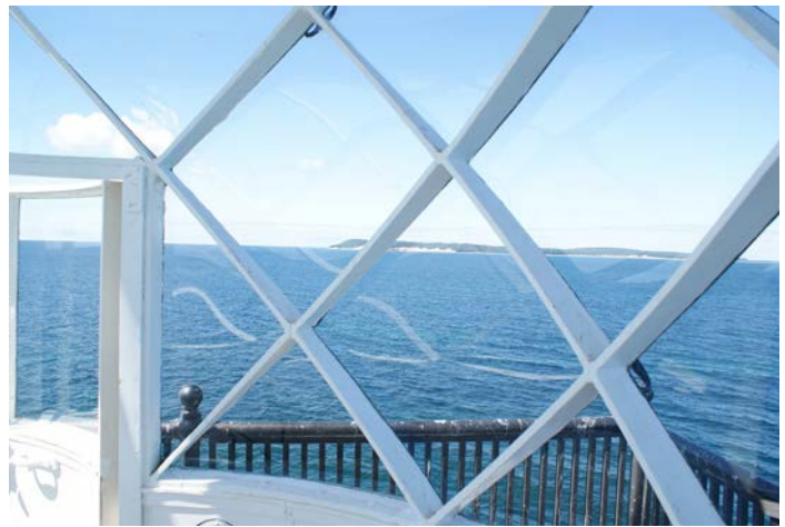
Figure 1D-127 Interior view of the curved metal mullions and glass in the Lantern.
