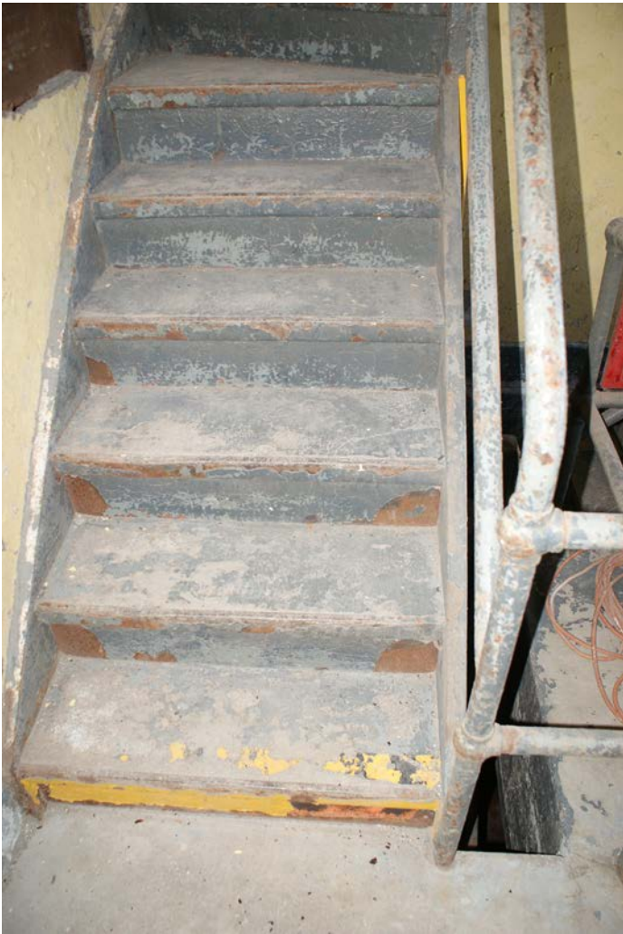
Figure 1D-184 Metal pan and concrete stair leading up to Level 2.
