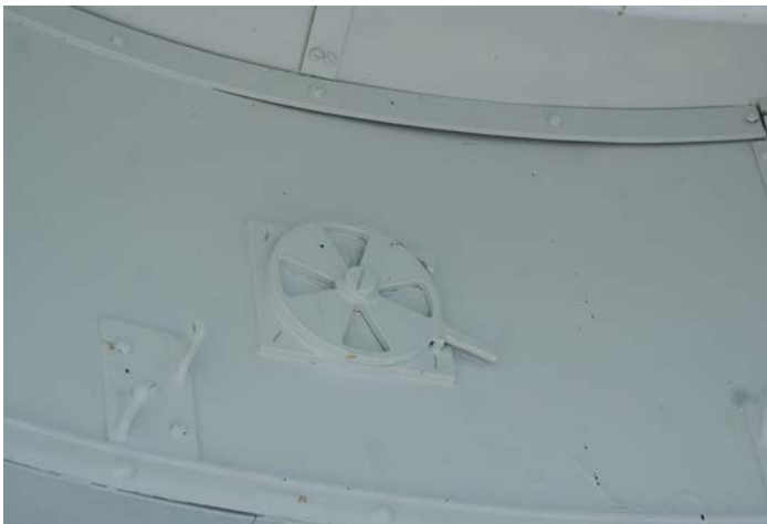
Figure 1D-126 Vents in upper walls of the Lantern
