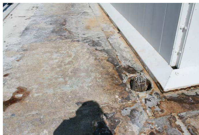
Figure 1D-14: Roof drain and corroded steel plate at the watch deck, Level L-3. Exterior curb with single anchor bolt at corner of tower is visible.
