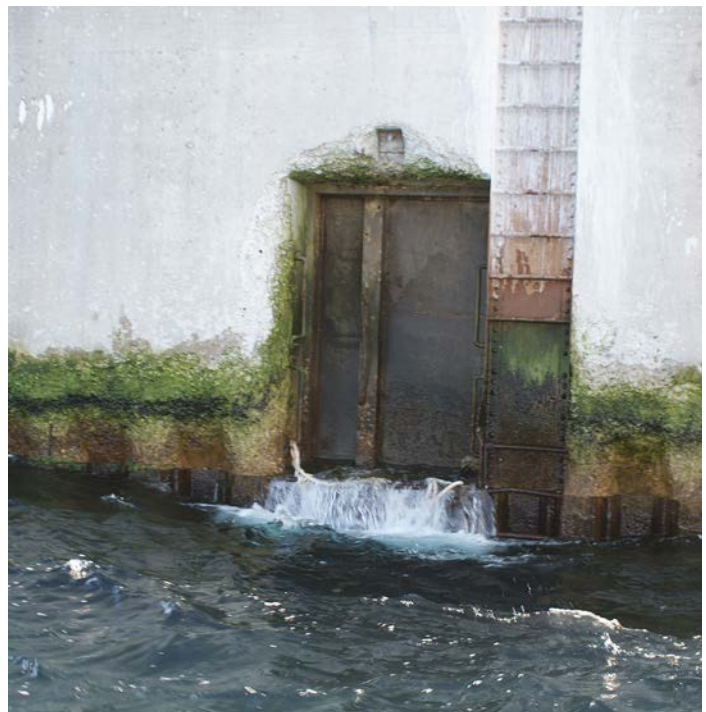
Figure 1D-72 Vertical steel ladder on the north wall next to the sea door. Two rungs are missing near the bottom.
