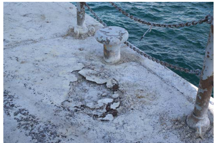
Figure 1D-76 View of the deteriorated surface of the steel plate on the Pier Deck.
