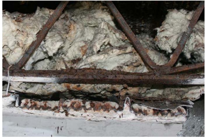
Figure 1D-48 Localized corrosion of metal bar joists.
