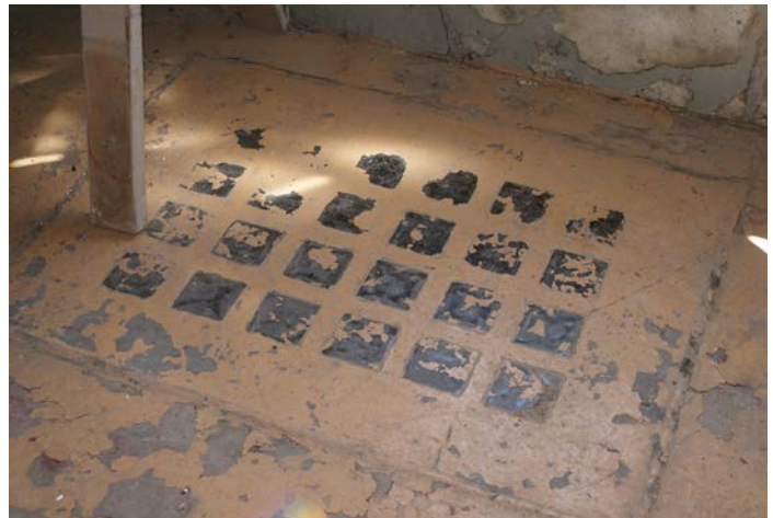
Figure 1D-162 Precast concrete and 24 glass block deck light as seen from Level 1.
