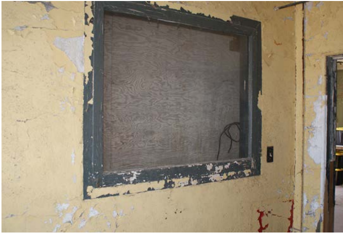
Figure 1D-175 Close-up view of the borrowed light at Level 1.
