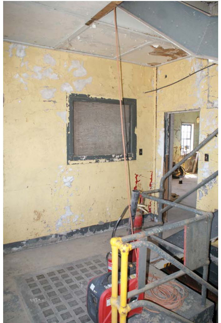
Figure 1D-173 View of borrowed light and partial view of deck light in the main entry room at Level 1.
