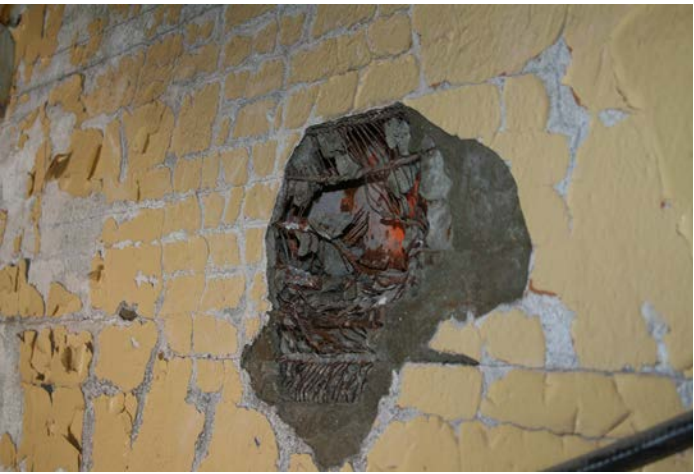
Figure 1D-28 Damaged plaster and lath in stairwell.
