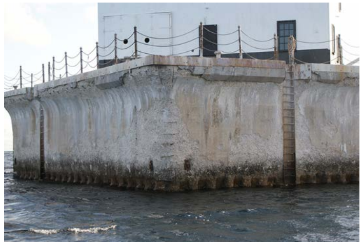
Figure 1D-70 Deteriorated concrete and exposed reinforcing bars on the southwest corner.
