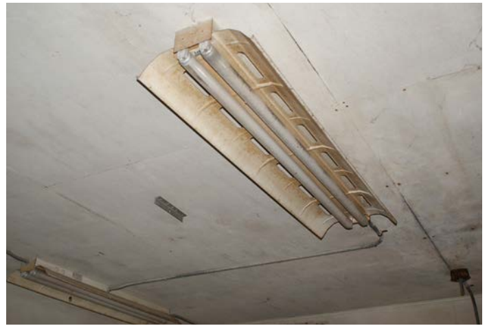
Figure 1D-234 Surface mounted fluorescent light fixture.
