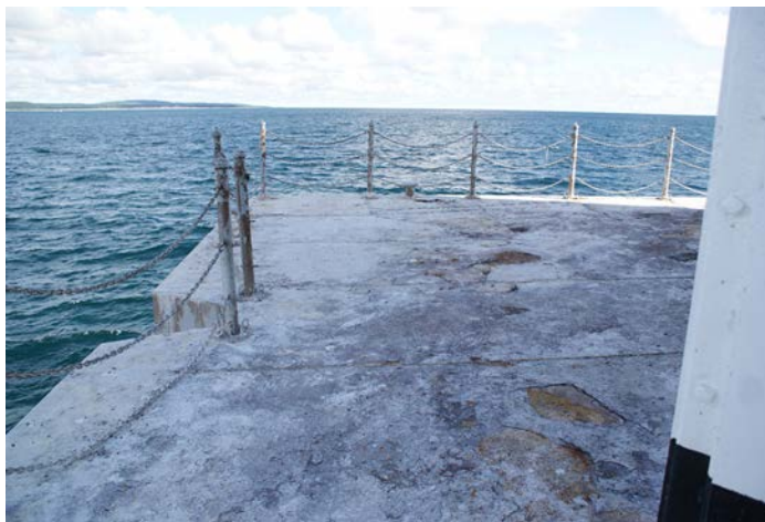
Figure 1D-75 View of the deteriorated surface of the steel plate on the Pier Deck.
