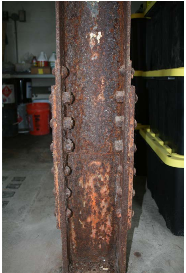
Figure 1D-37 Column splice of southernmost interior column at pier deck, Level L-1. Note riveted connection at bottom and through-bolted connections at top of splice plates. Extra rivet at top of connection for splice plate to accommodate change in flange thickness of columns.
