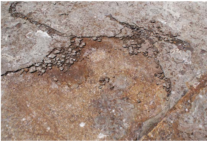
Figure 1D-92 Deteriorated surface condition of the steel deck plate at the Watch Deck.
