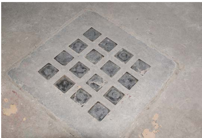
Figure 1D-165 Smaller deck light with 16 glass blocks.
