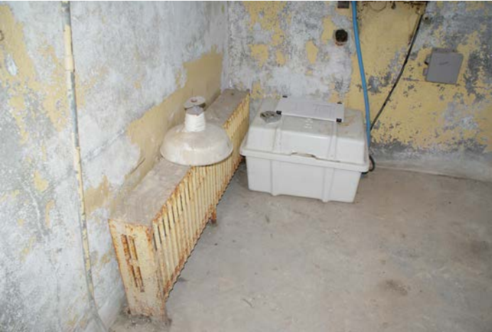
Figure 1D-240 Abandoned cast iron radiator located on tower Level 5.
