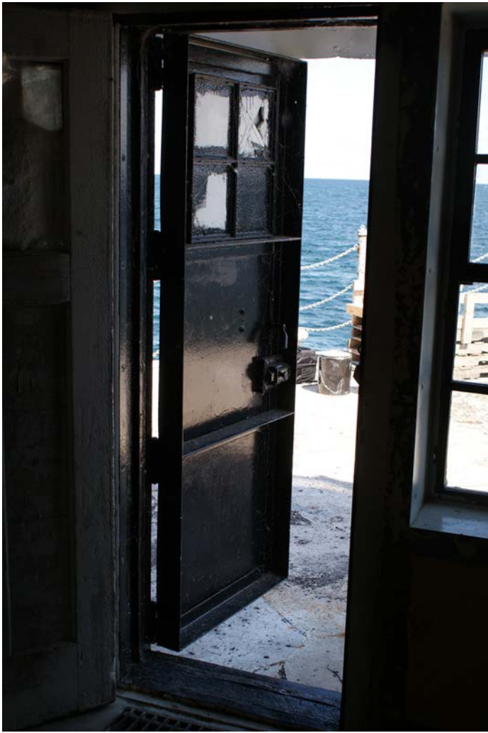
Figure 1D-110 Exterior, out-swinging metal door at entry from the Pier Deck.
