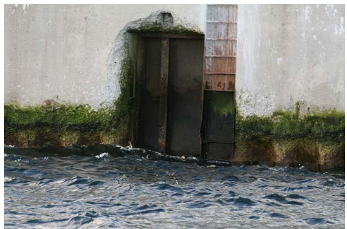
Figure 1D-04: Water level steel access door on north side of concrete crib. Note spalling of concrete around opening and heavy organic growth above the water. The top of the steel sheet piling is visible on the right side of the photo at the water level. The steel ladder is missing
