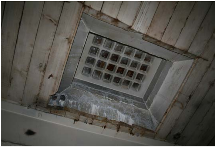
Figure 1D-35 Craze cracking and staining of concrete at glass skylight opening in pier deck, Level L-1 floor structure.
