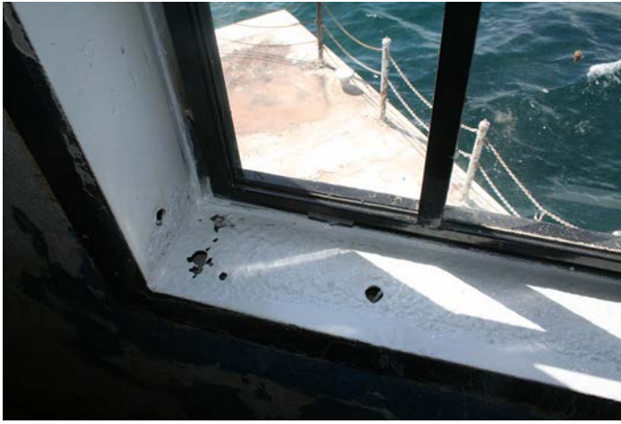
Figure 1D-33 Pitted and section loss of steel angle window framing.
