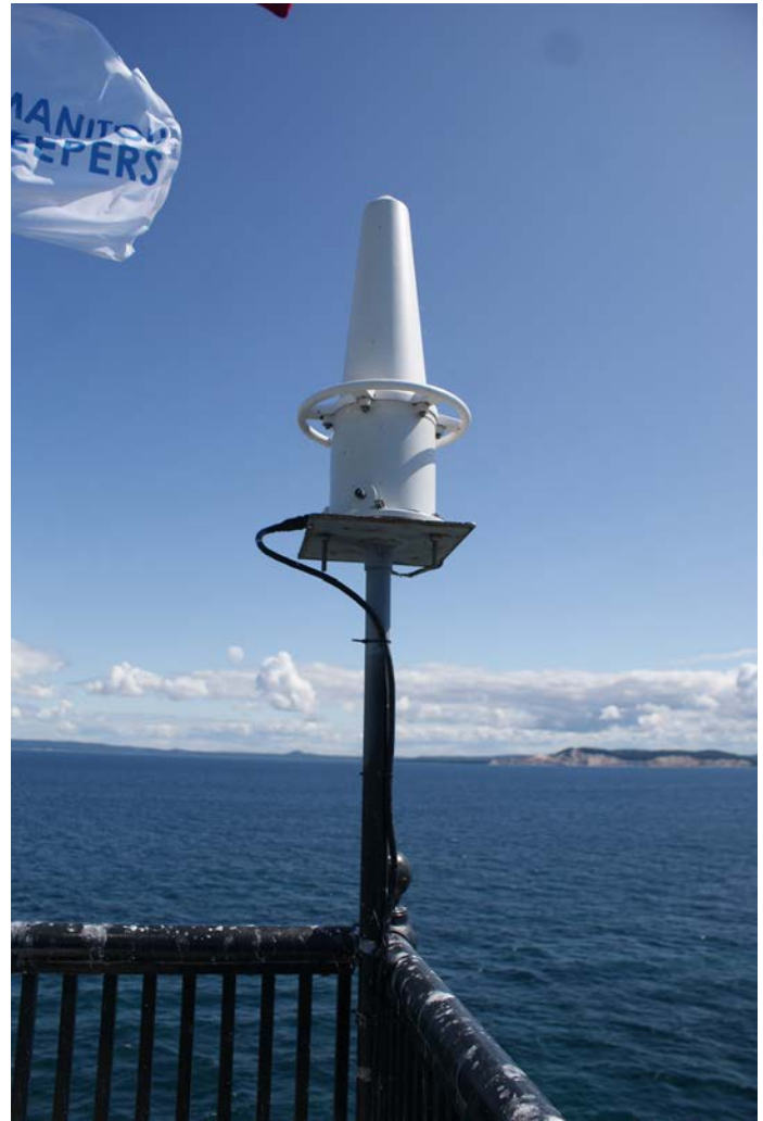
Figure 1D-141 Radar unit secured to the metal guardrail.
