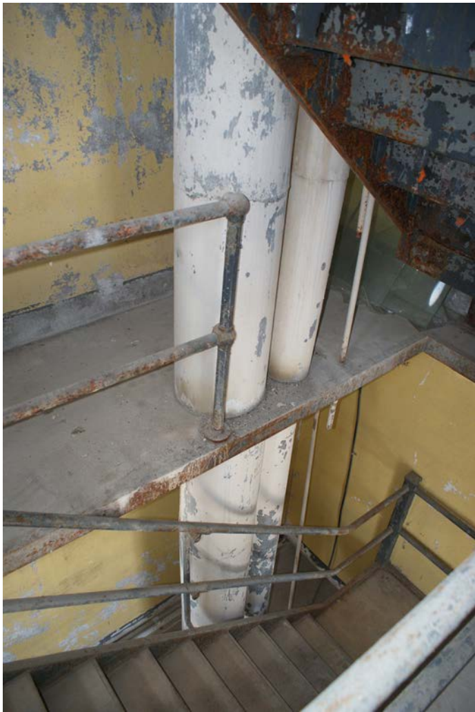
Figure 1D-218 Metal chimney pipes passing through Level 4.
