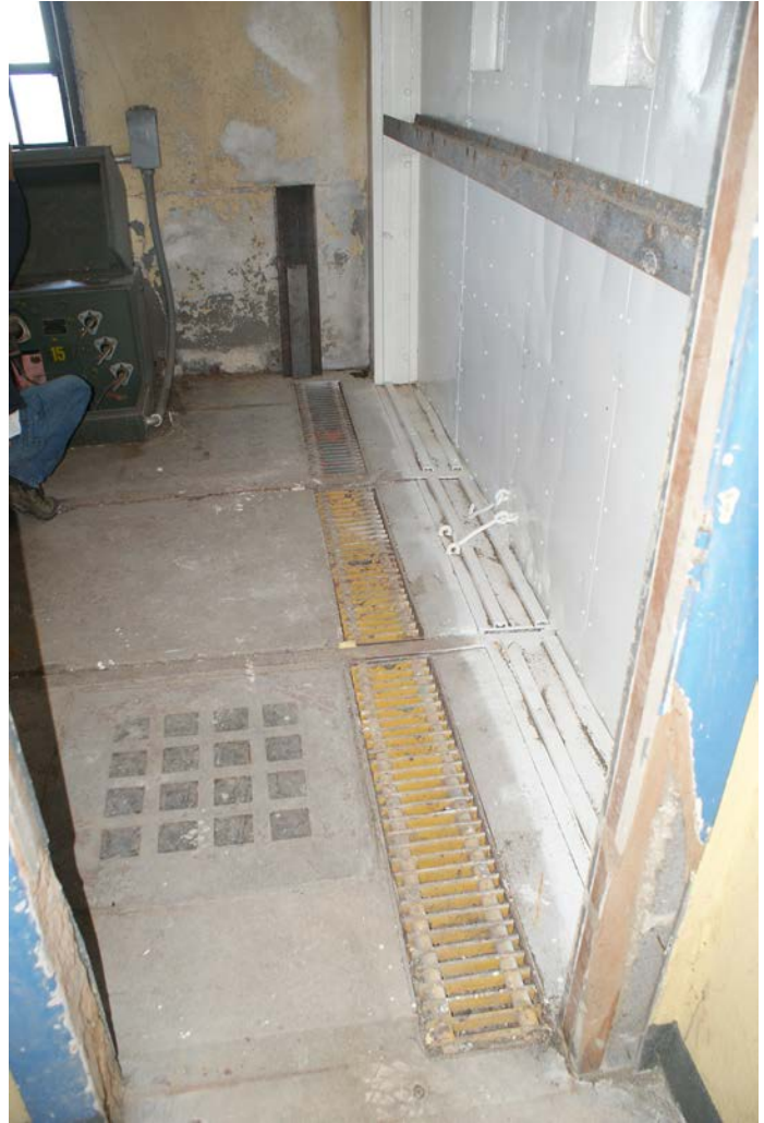
Figure 1D-170 Trench drain across the Boat Room door opening with adjacent deck light.
