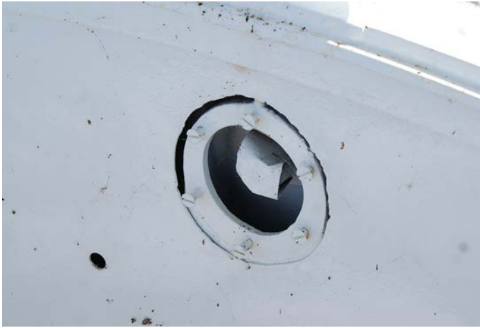
Figure 1D-124 Vent opening in the Lantern wall. The vent cover is missing.
