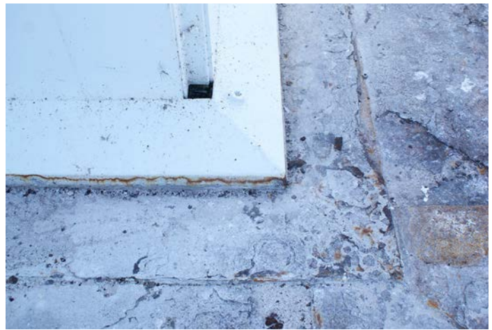
Figure 1D-93 Deteriorated surface condition of the steel deck plate at the Watch Deck.
