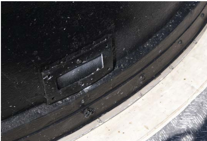
Figure 1D-135 Ventilation opening at base of Lantern.
