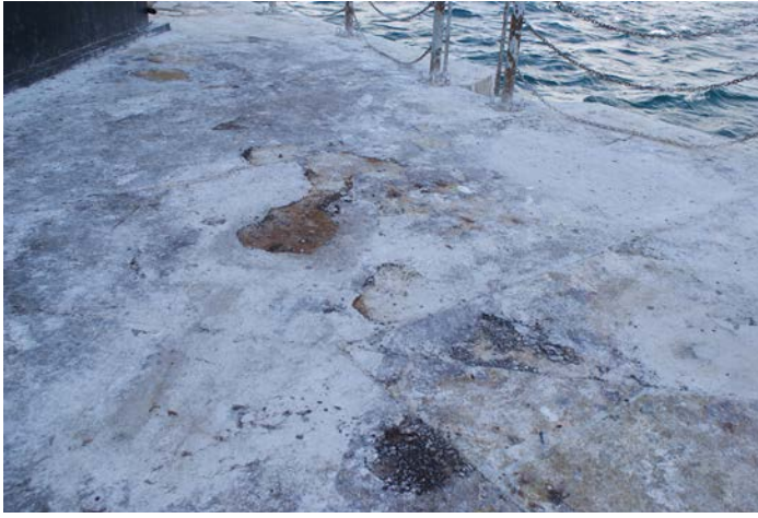
Figure 1D-77 View of the deteriorated surface of the steel plate on the Pier Deck.
