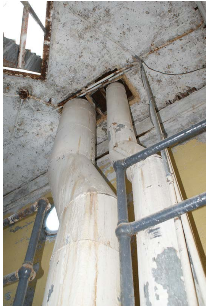
Figure 1D-220 Metal chimney pipes terminating at the underside of the Lantern Deck.
