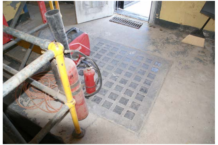
Figure 1D-164 Large deck light adjacent to the main entry door at Level 1.
