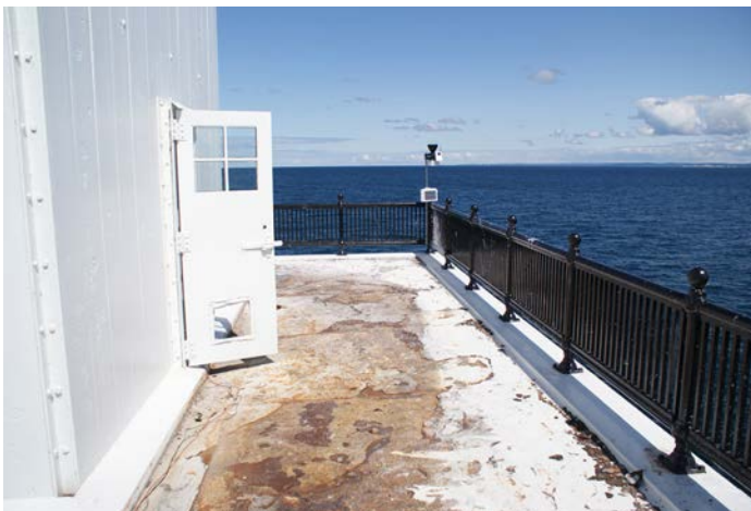
Figure 1D-88 View of the steel plate deck surface at the Watch Deck, Level 3.
