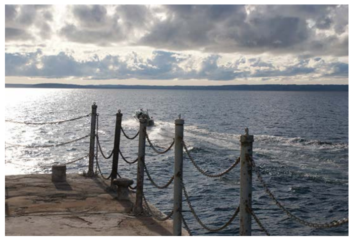
Figure 1D-80 Steel pipe posts and chain link guardrail at the perimeter of the Pier Deck.
