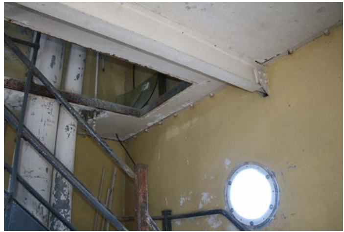
Figure 1D-55 Typical center steel beam of floor structures of upper levels of tower.
