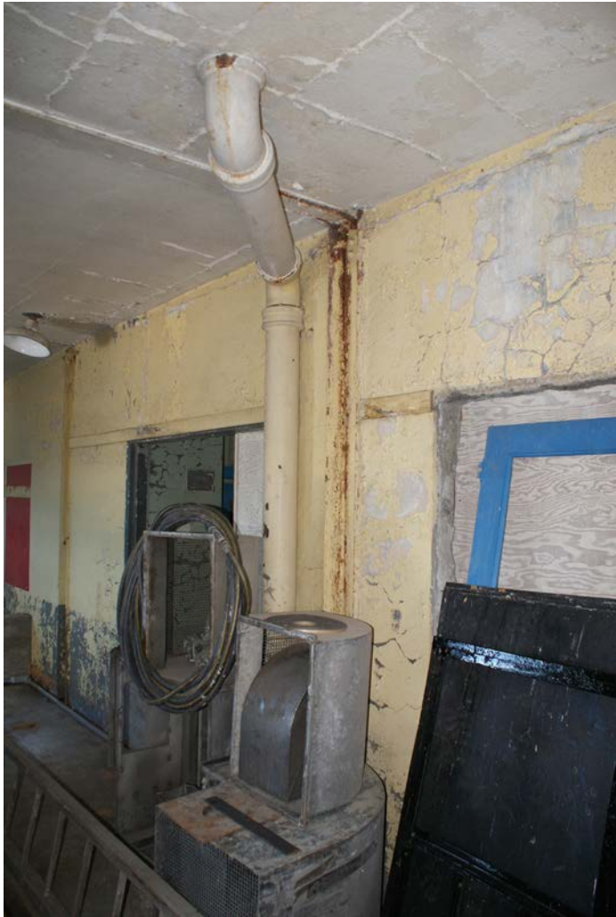
Figure 1D-239 Cast iron roof drain line exposed in the Boat Room on Level 1.
