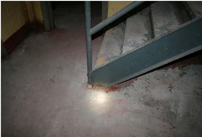
Figure 1D-59 Minor corrosion of stair stringer at basement level.
