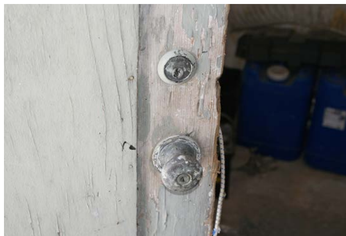
Figure 1D-120 Door hardware on the in-swinging wood door.
