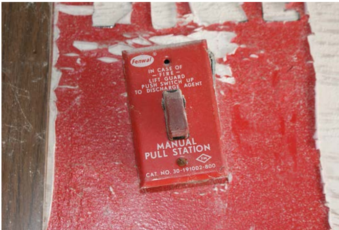
Figure 1D-246 Fire alarm pull station located on Level 1.
