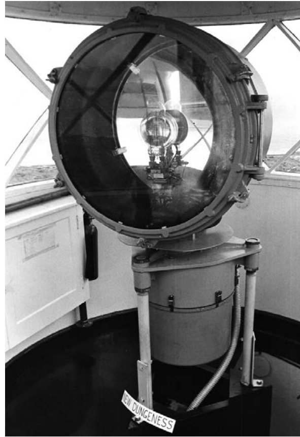
Figure 1A-08: Photo of the single DCB-24 aero beacon installed in the New Dungeness Lighthouse in Sequim, Washington in 1976.
