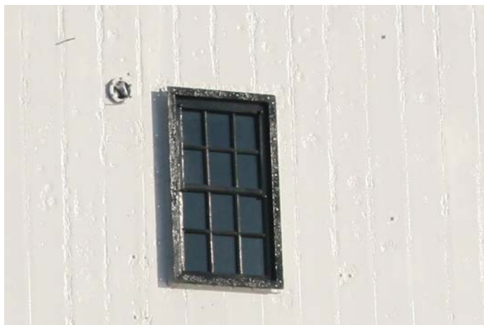
Figure 1D-13: Pitted exterior surfaces of the wall channels and window angle frame.
