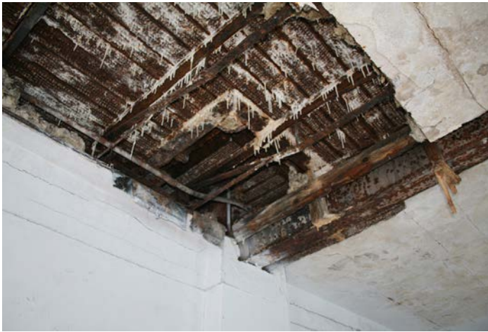
Figure 1D-49 Upper tower wall framing bearing on watch deck, Level L-3, structure. Note water staining of wood furring, corrosion of steel, and stalactites.
