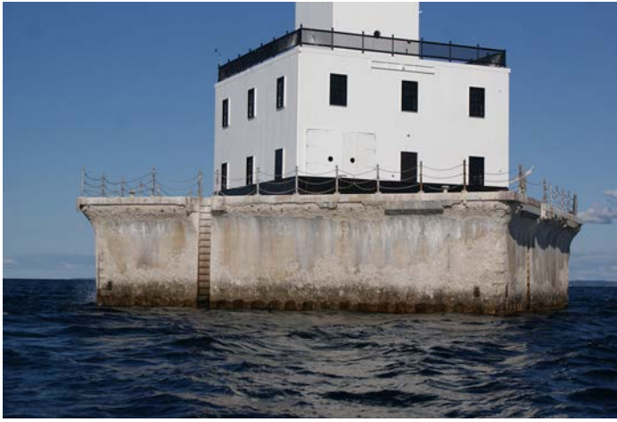
Figure 1D-64 West face of the concrete crib.
