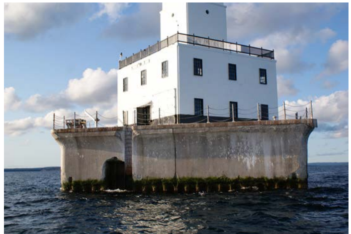
Figure 1D-62 North face of the concrete crib.
