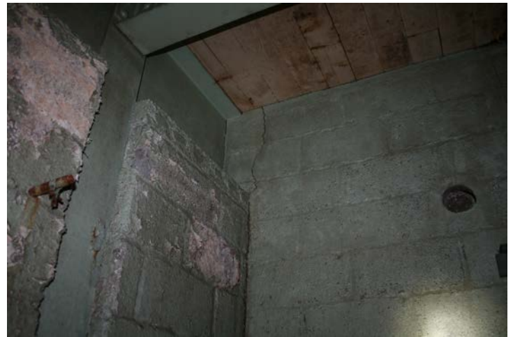
Figure A-2 Exterior steel column of tower within the basement wall.
