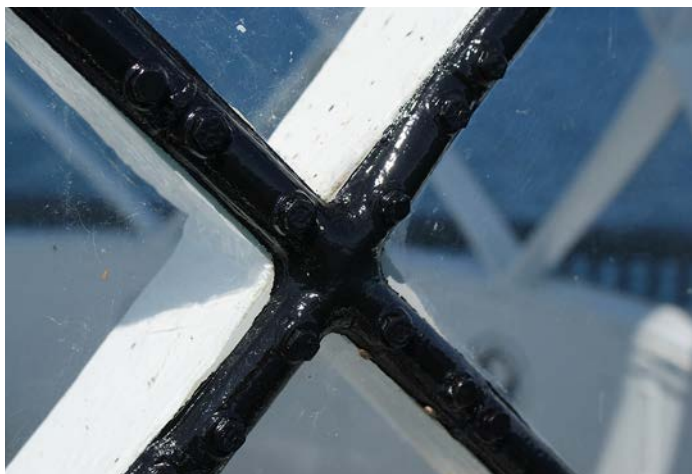
Figure 1D-131 Exterior view of glazing mullion covers.
