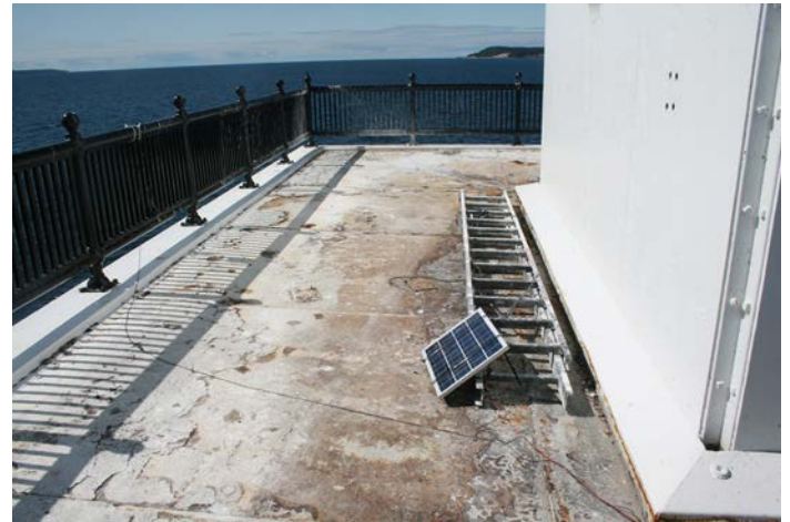
Figure 1D-17 Corroded steel plates on exterior surface of watch deck, Level L-3. Exterior curb with single anchor bolt at corner of tower is visible.
