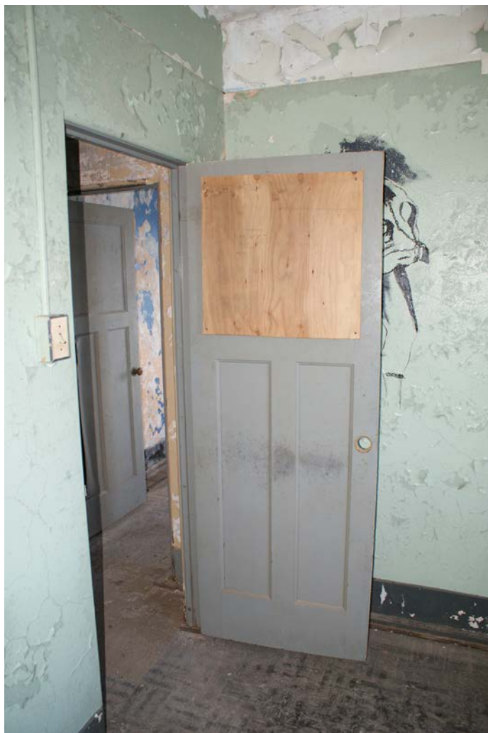
Figure 1D-195 Two-panel wood door with glass light at Office on Level 2.
