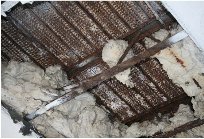
Figure 1D-47 Corroded metal bar joists.
