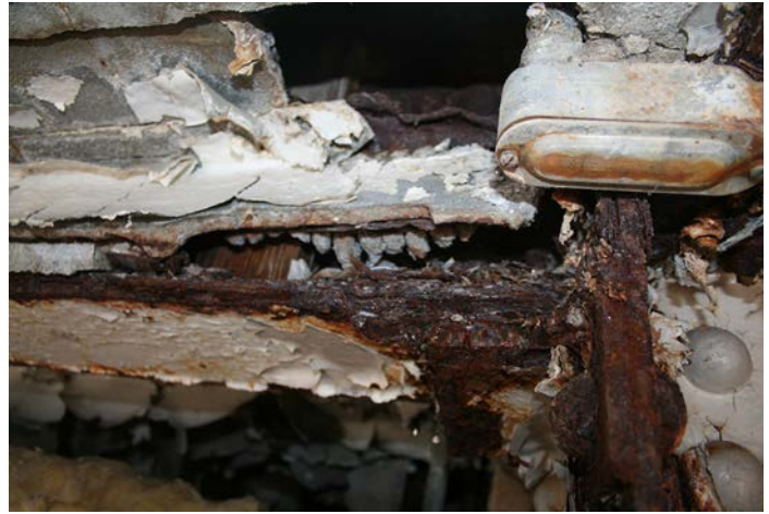
Figure 1D-40 Significant corrosion of steel flanges of beams and columns at second floor structure, Level L-2, at southernmost interior column.
