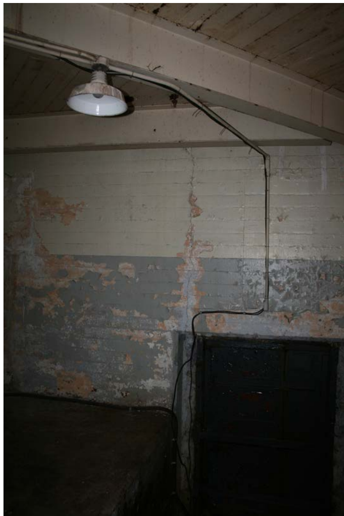
Figure 1D-22: Vertical crack in interior surface of the concrete crib wall at west end of water level access door.
