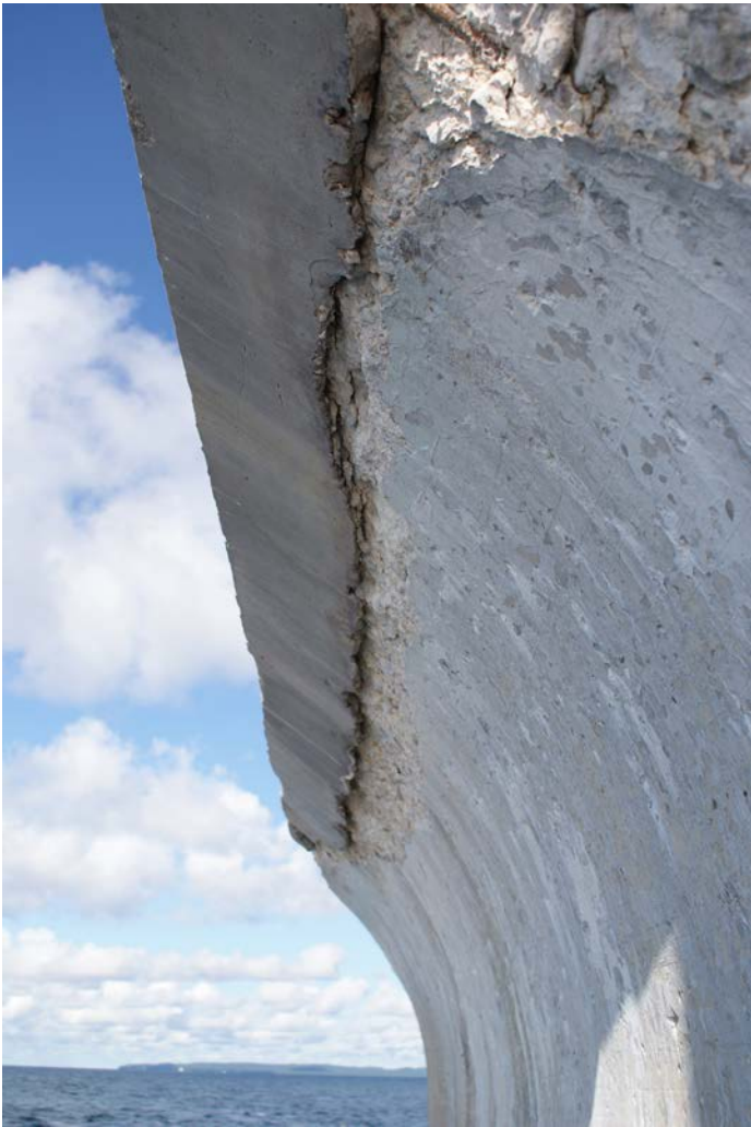
Figure 1D-68 Concrete repair at wave edge.
