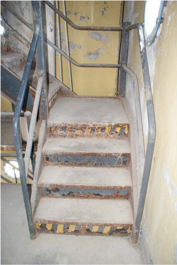
Figure 1D-215 View of metal pan and concrete stairway at Level 4.
