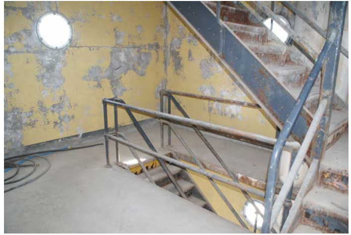
Figure 1D-216 Stairway and steel pipe guardrails around stair opening at Level 4.
