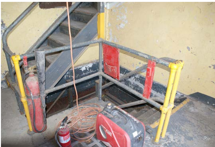
Figure 1D-174 View of the open stairway at Level 1 showing the steel pipe guardrail.
