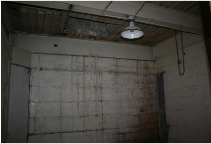
Figure 1D-20 Steel beam and CMU wall construction visible in basement. Note water staining on CMU walls and skylight opening in ceiling. Note vertical crack between chamfered concrete corner and CMU wall.
