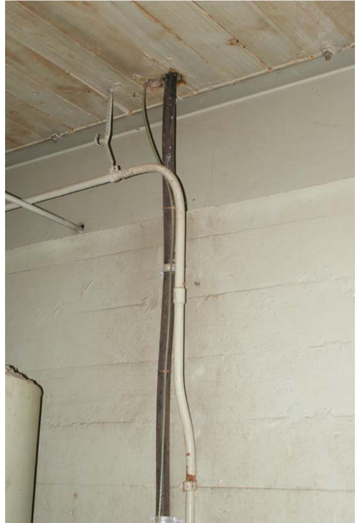
Figure 1D-227 Main electric cable running up the wall in the Basement Water Room.
