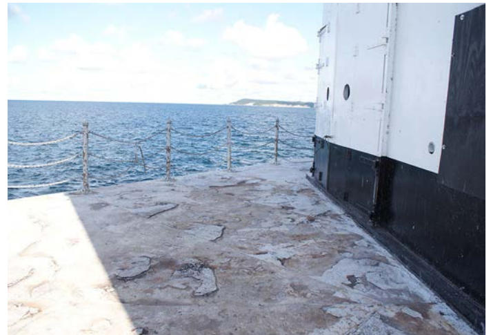
Figure 1D-74 View of the deteriorated surface of the steel plate on the Pier Deck.
