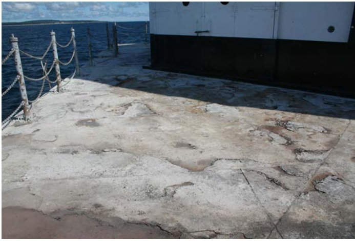
Figure 1D-08: Corroded steel plates on exterior surface of pier deck, Level L-1.
