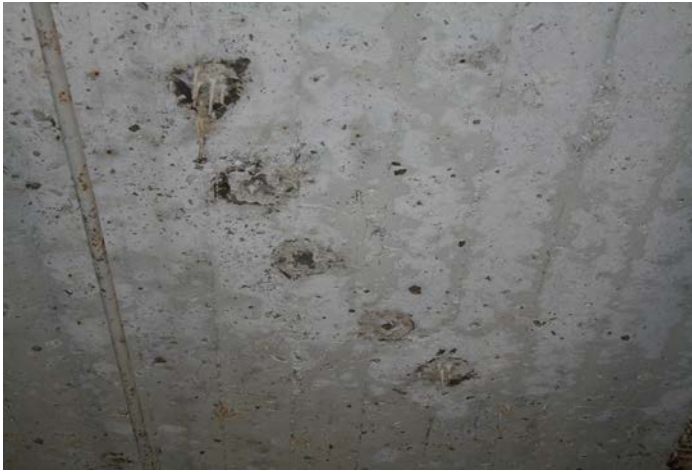
Figure 1D-58 Stalactites on underside of lantern deck concrete slab at location of lantern anchorage.
