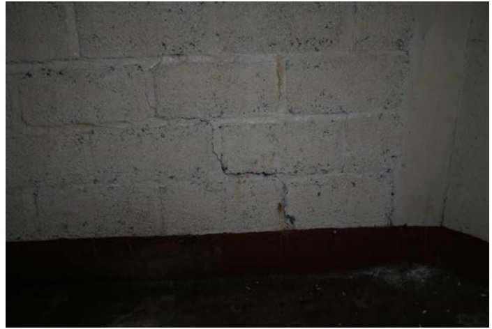
Figure 1D-23 Step cracking at base of CMU wall.
