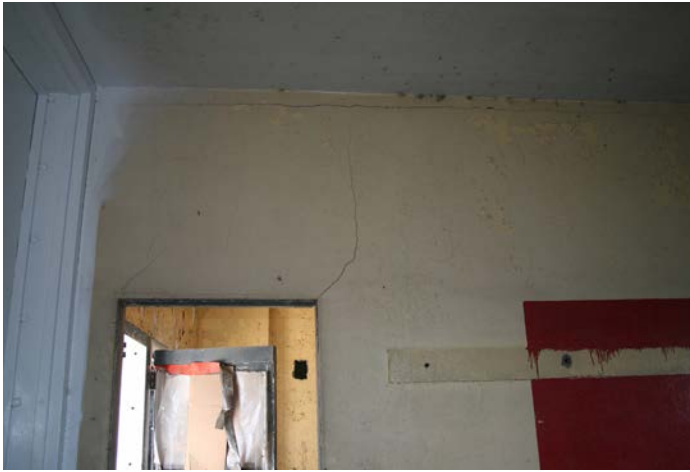
Figure 1D-29 Cracking in plaster at right side of door from boat room to entry. Note horizontal crack at top of wall near ceiling.
