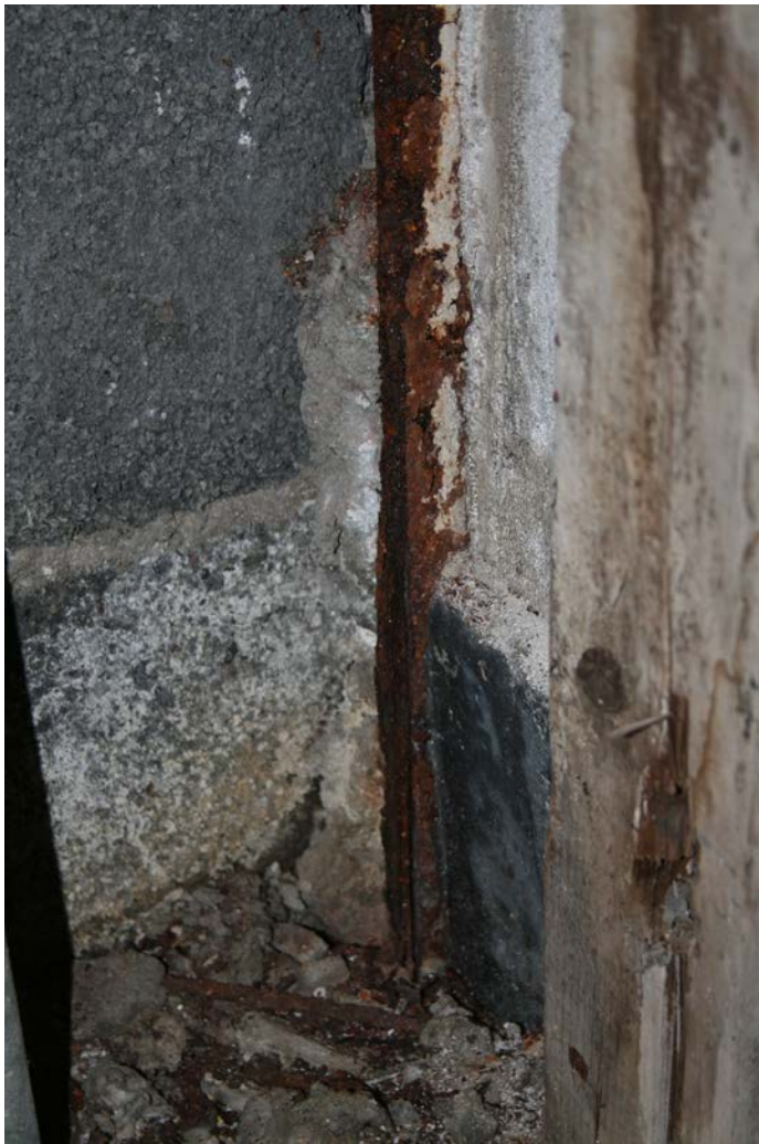
Figure 1D-43 Corroded at warped flange at southernmost interior column. Note portions of the steel column are on debris on top of floor.
