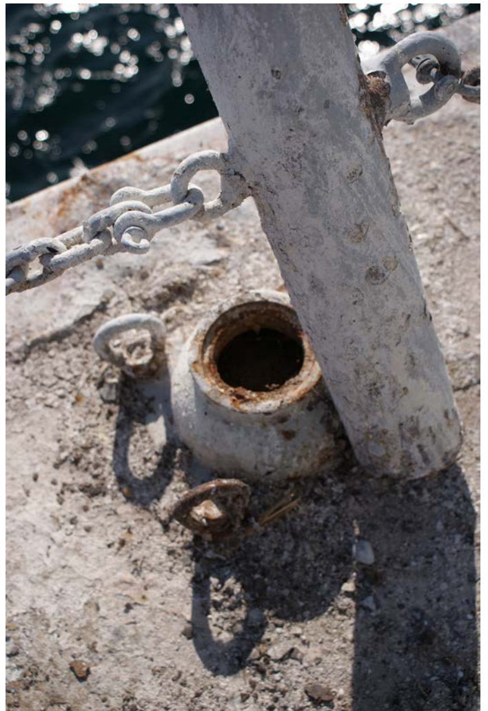
Figure 1D-83 View of damaged guardrail post broken from the base.
