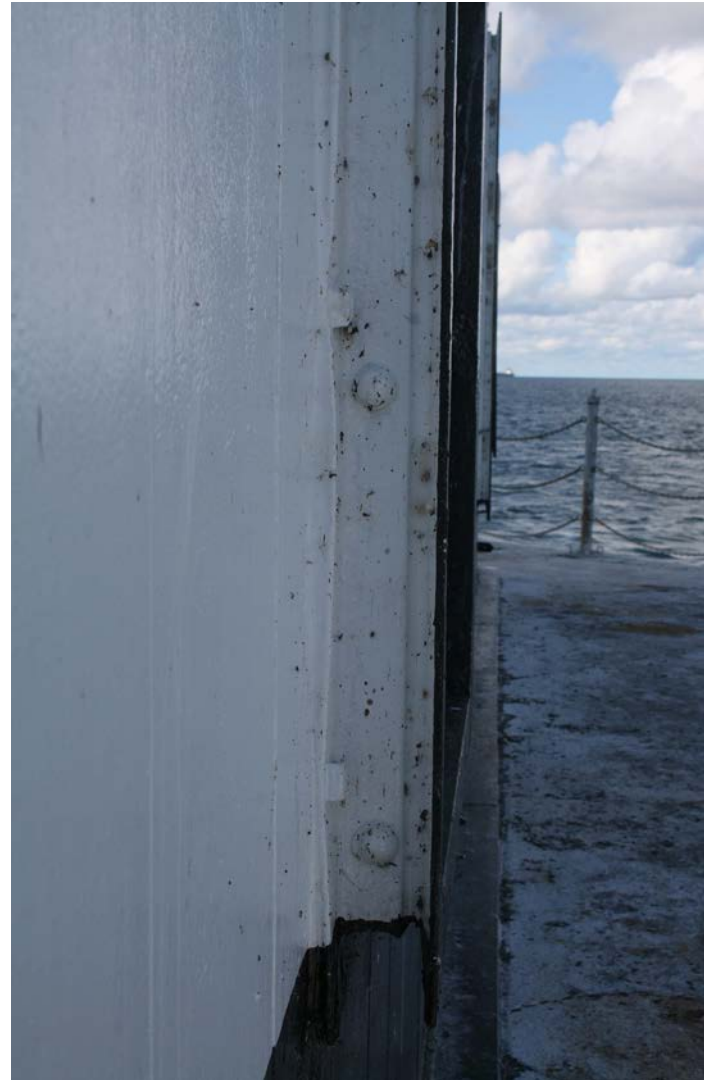
Figure 1D-11: Warped steel leg of angle at window framing bolted to wall structure related to corrosion of the steel in this area.
