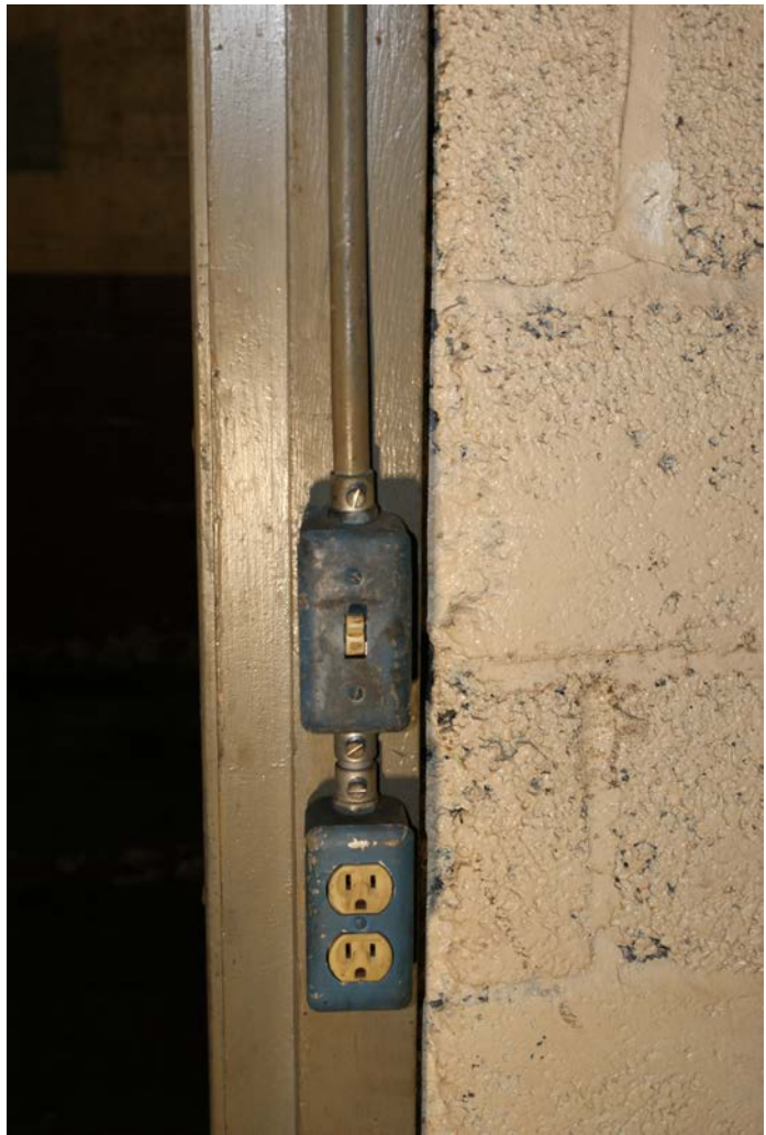
Figure 1D-232 Typical surface mounted electrical devices.
