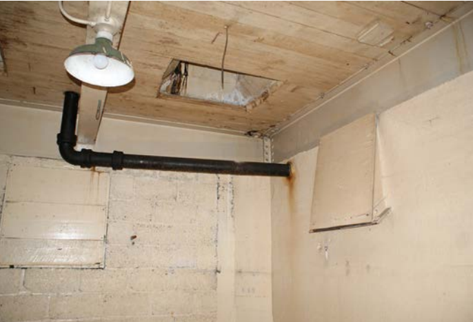
Figure 1D-238 Cast iron sanitary waste line exposed in the Basement.
