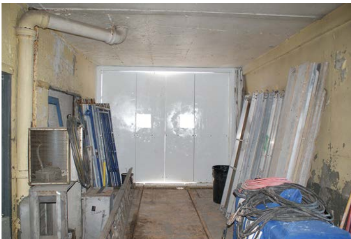
Figure 1D-171 View of the steel angle boat rails in the floor of the Boat Room.
