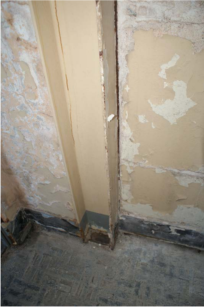
Figure 1D-204 View of exposed steel column on Level 2 and poor interior finishes.
