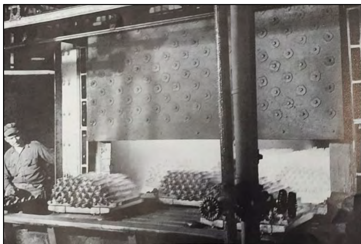
Image 10: Steel Tank Treads Leaving Furnace at Campbell, Wyant, & Cannon, c.1945 (CWC-Textron)
