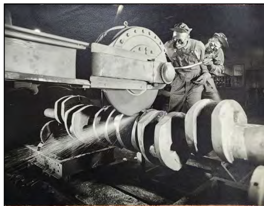
Image 16: African American Workers Clean a Crankshaft at Campbell, Wyant, & Cannon Foundry, c.1945 (CWC-Textron)
