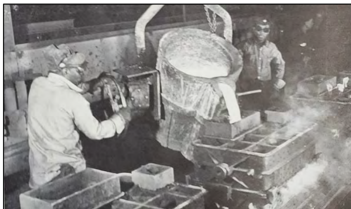
Image 11: African American Workers Pour Cylinder Blocks at Campbell, Wyant, & Cannon, c.1945 (CWC-Textron)
