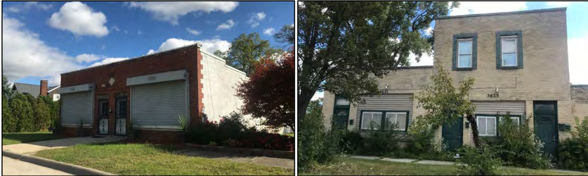
Image 33. At left is the commercial building at 3829 Harrison, at right is the commercial buildings at 3621-3625 Harrison. (Kraemer Design Group 2022)
