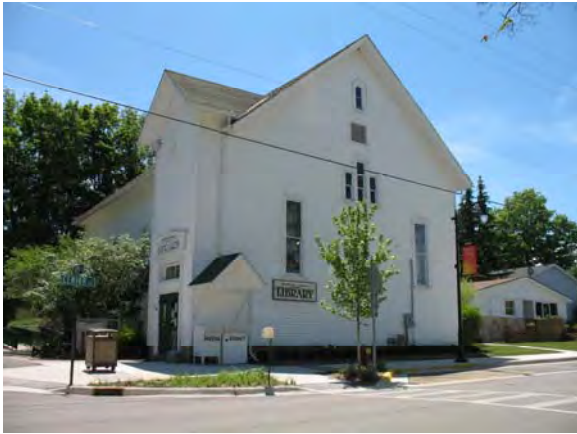
137 Center Avenue, Douglas Saugatuck Douglas Library
