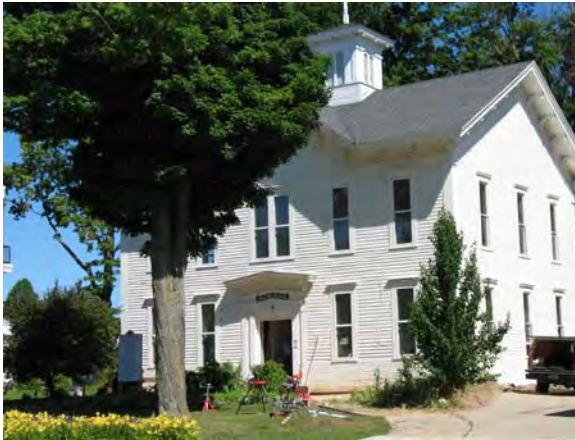
Center Avenue, Douglas Douglas Union School
